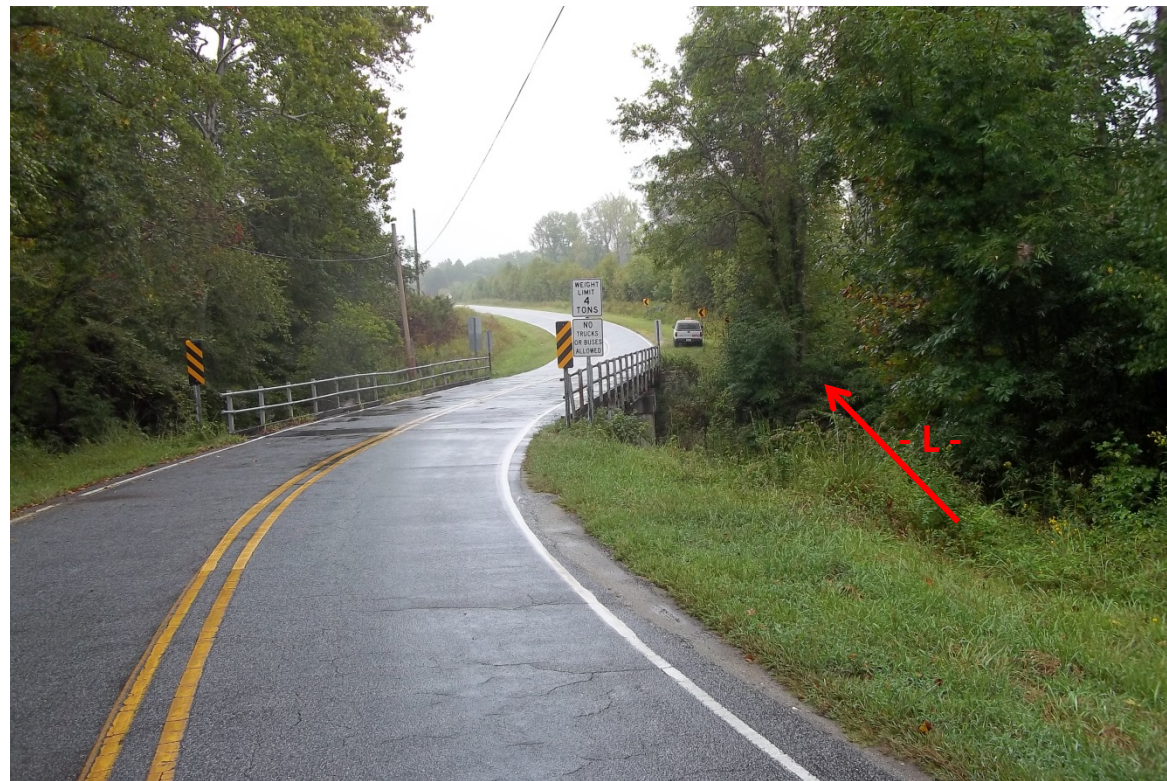
Photograph No. 2: View of existing bridge looking east
