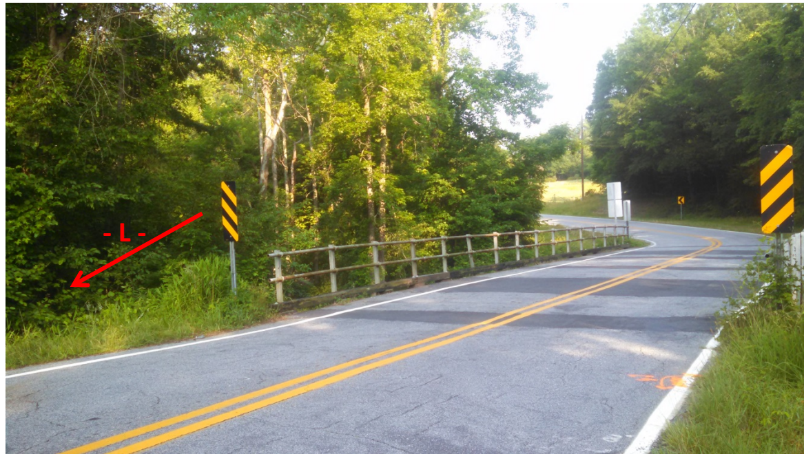
Photograph No. 1: View of existing bridge looking west
