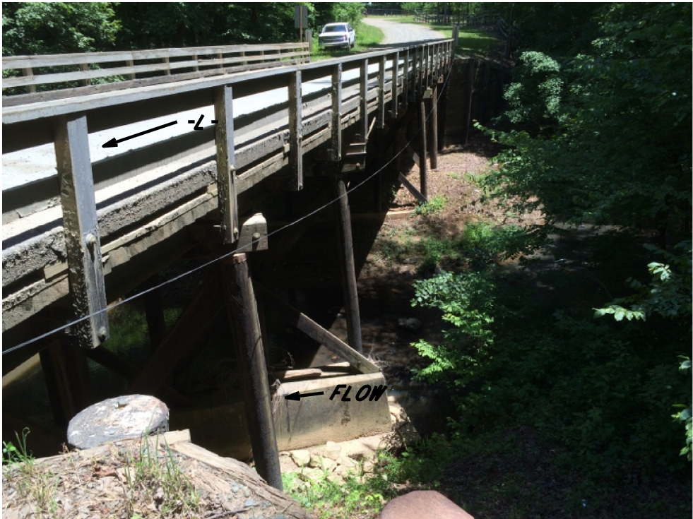
PHOTOGRAPH 2: VIEW ALONG SOUTH SIDE OF BRIDGE I25 LOOKING SOUTHEAST.
