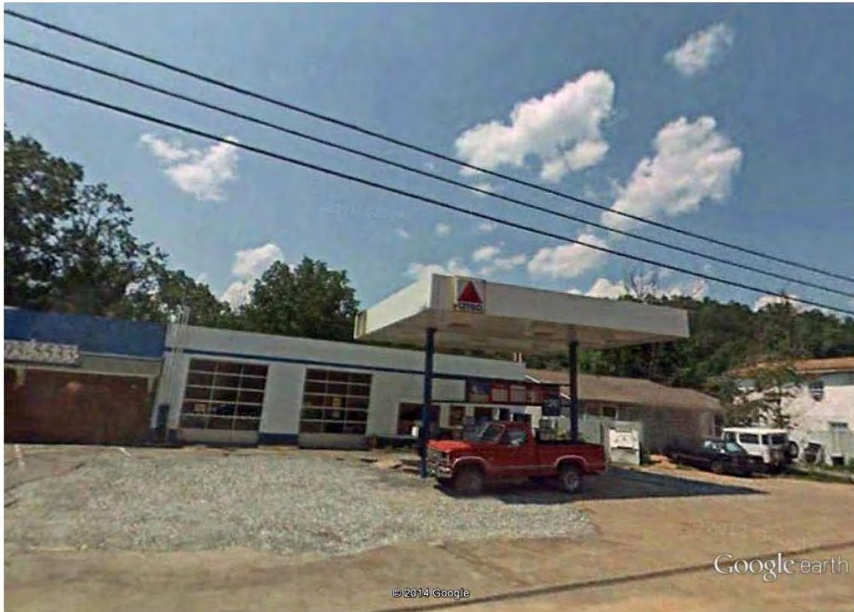
Photograph 1 : View looking west from Old Cullowhee Road at former service station on Parcel 013 in July 2008. Stone-covered areas to the north and south of former pump island are believed to be excavations associated with removal of former USTs and/or soil remediation. Service station does not appear to be operating at the time photo was taken.
