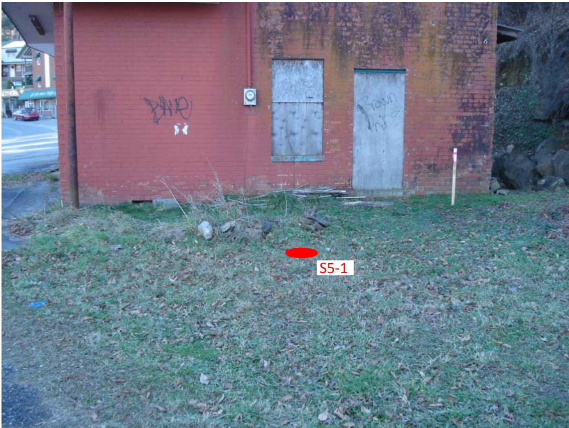
Photograph 1 : View looking south at soil boring location S5-1 at Parcel 005.
