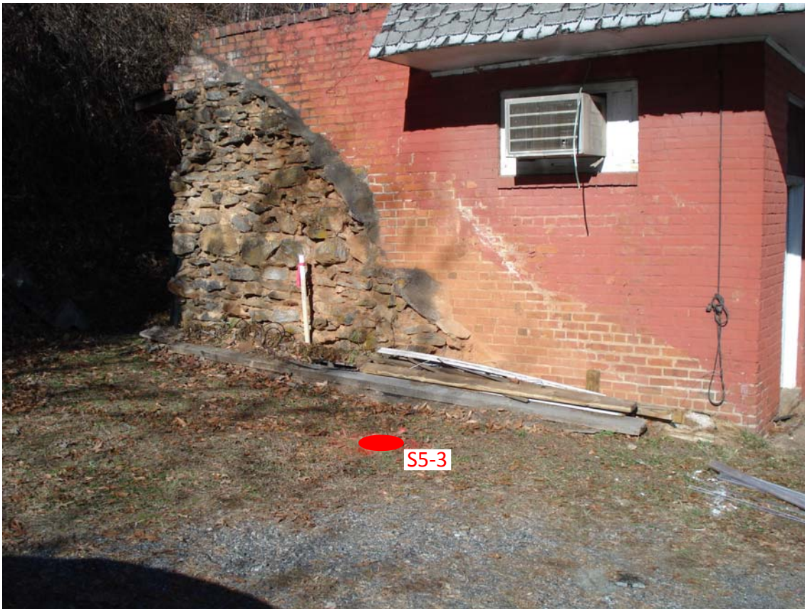
Photograph 3 : View looking northwest at soil boring location S5-3 at Parcel 005.
