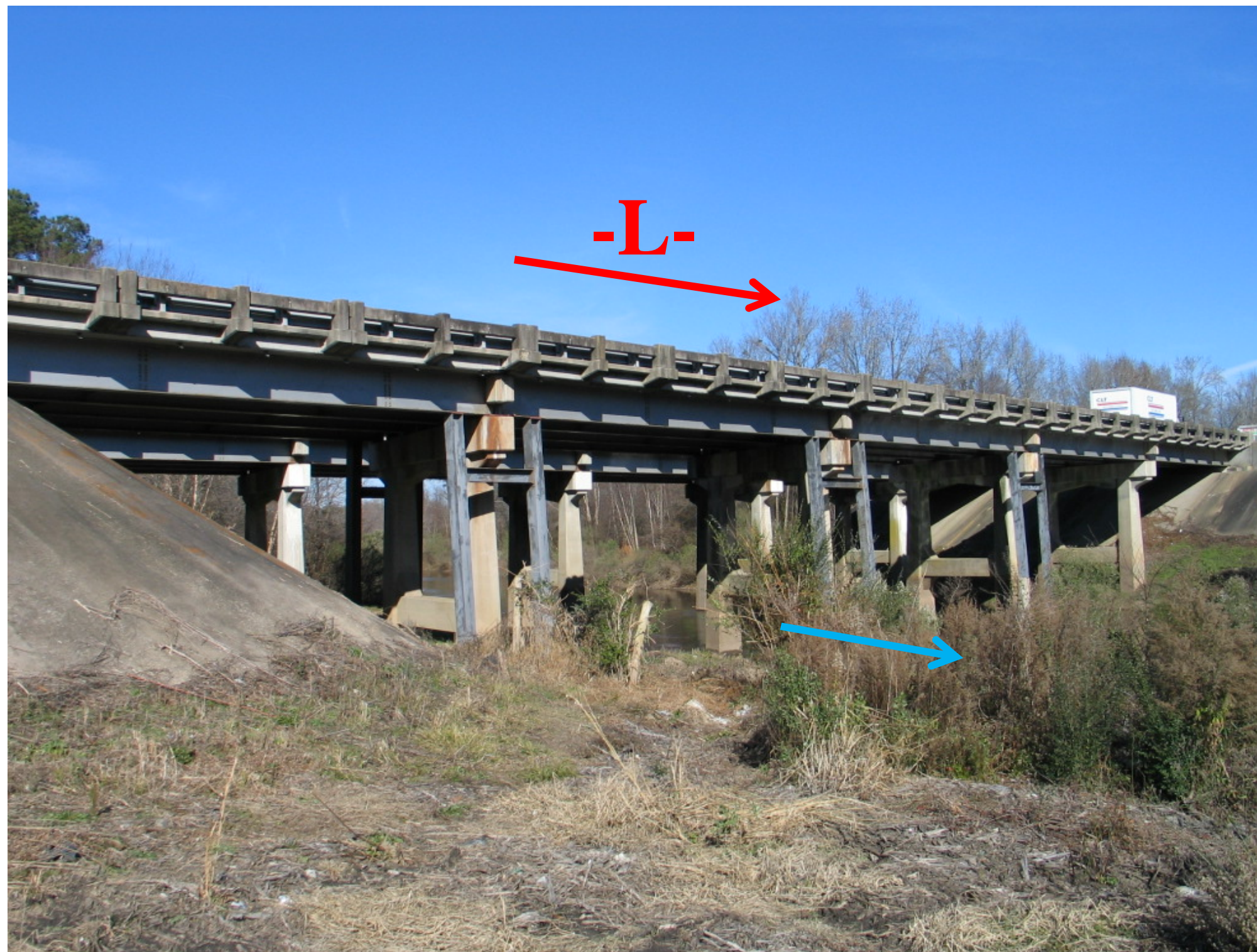
Looking North and upstream at Bridge No. 114
