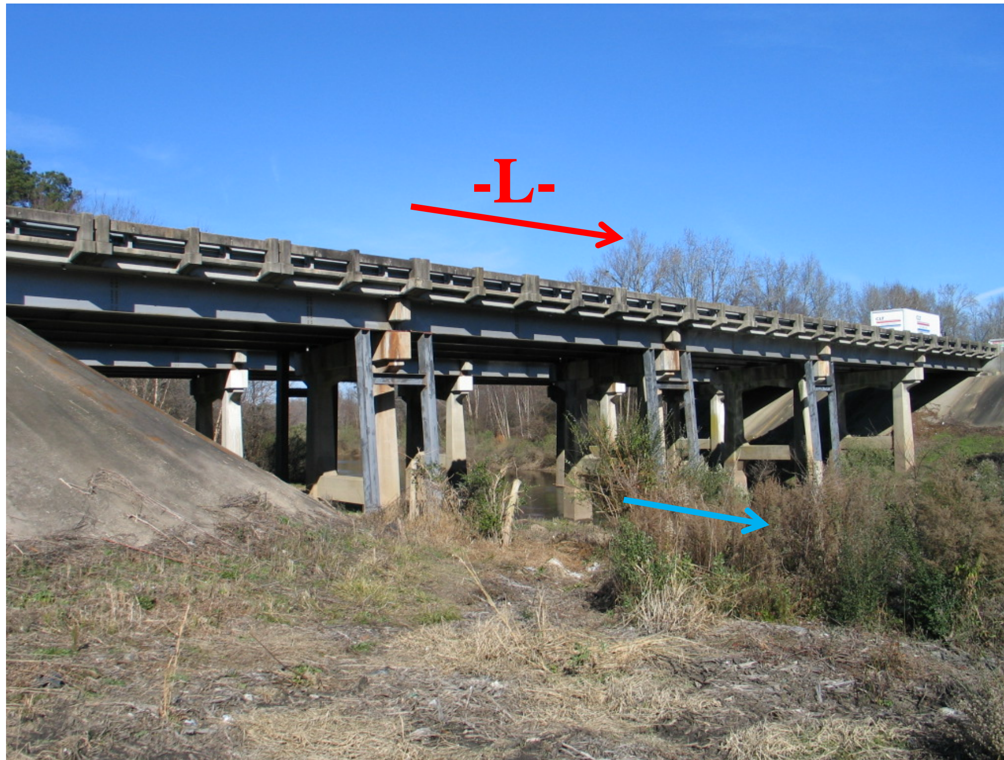
Looking North and upstream at Bridge No. 114
