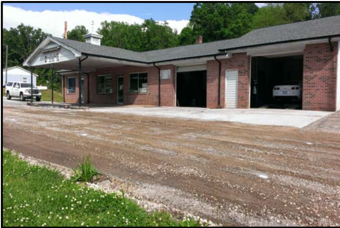
Photograph of On-Site Building (Facing Approximately Southeast)
