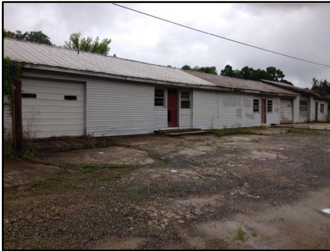
Photograph of Abandoned On-Site Building (Facing Approximately North)
