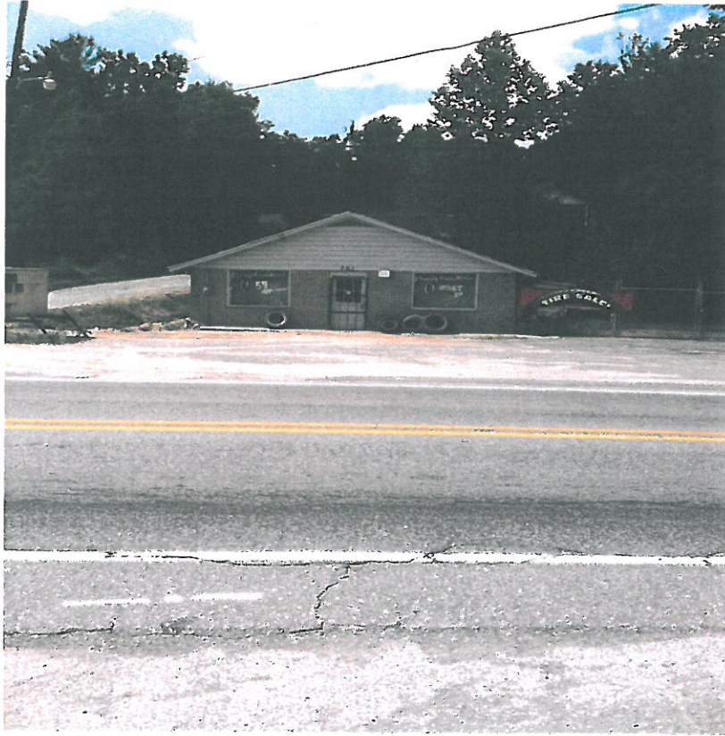
Photograph 1 – View of the used tire sales located on the western portion of the property.
