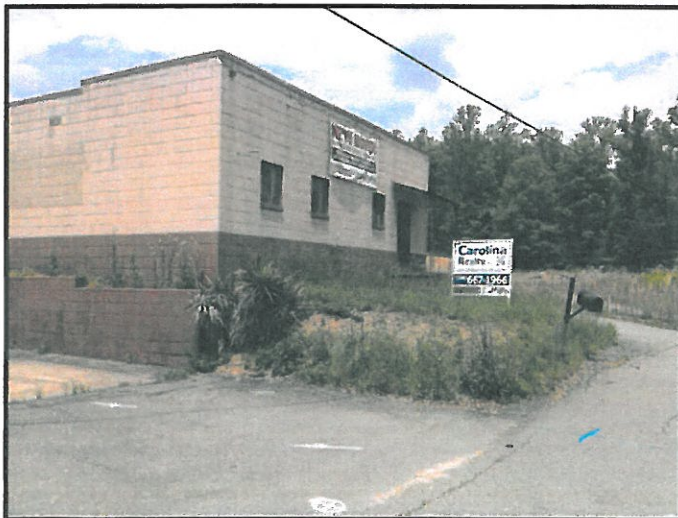
View of Print Building (Photograph Facing Approximately Northeast)
