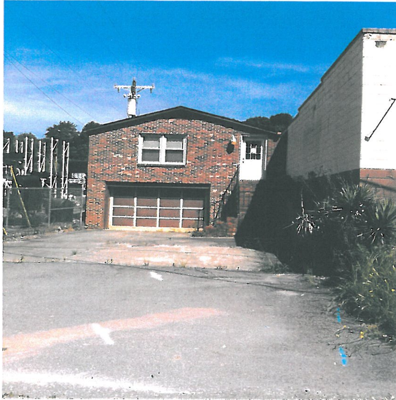
Photograph 3 – View of the residential portion of the structure.
