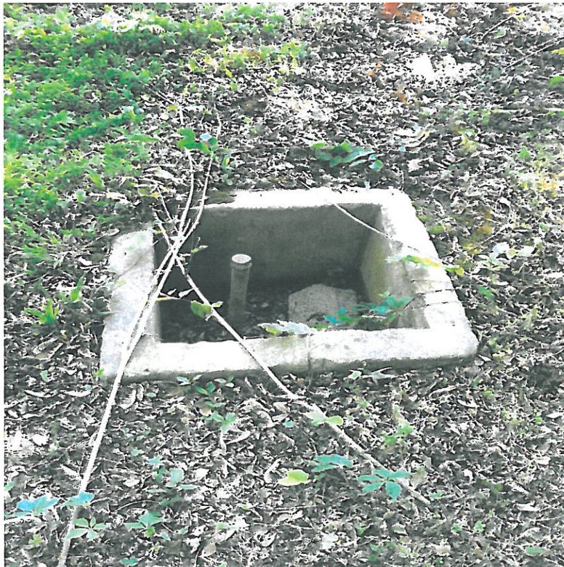
Photograph 8 – View of a vault and pipe observed north of the structure.
