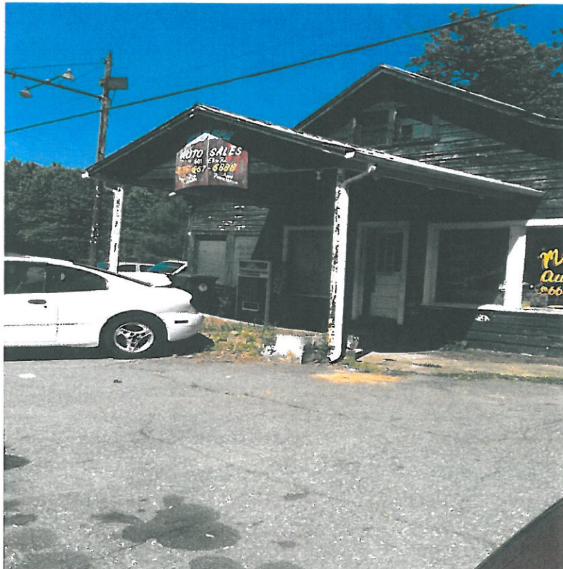
Photograph 4 – View of the front of the structure.
