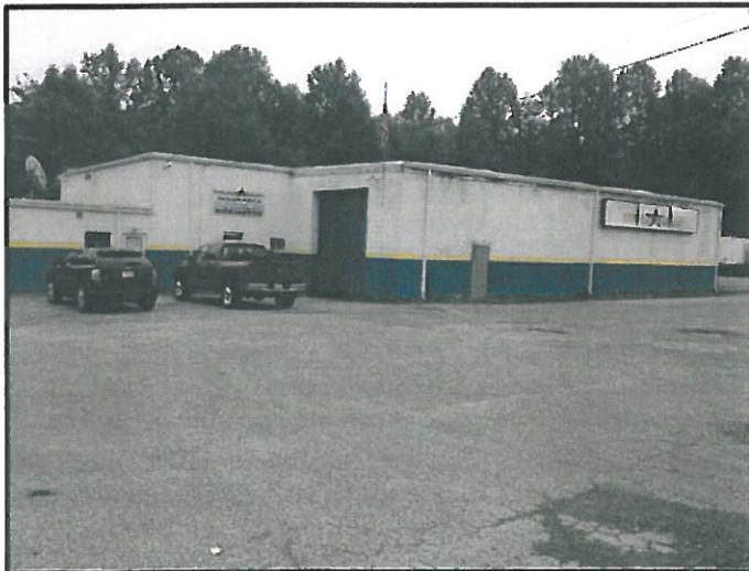
View of Truck Service Building (Photograph Facing Approximately Southwest)
