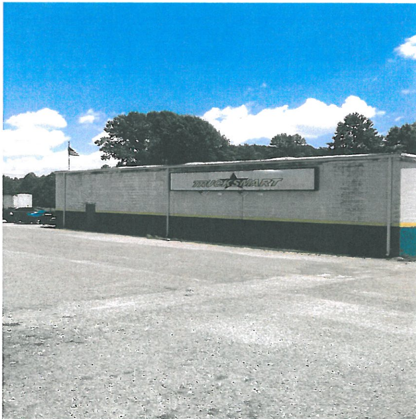
Photograph 2 – View of the northern portion of the structure.
