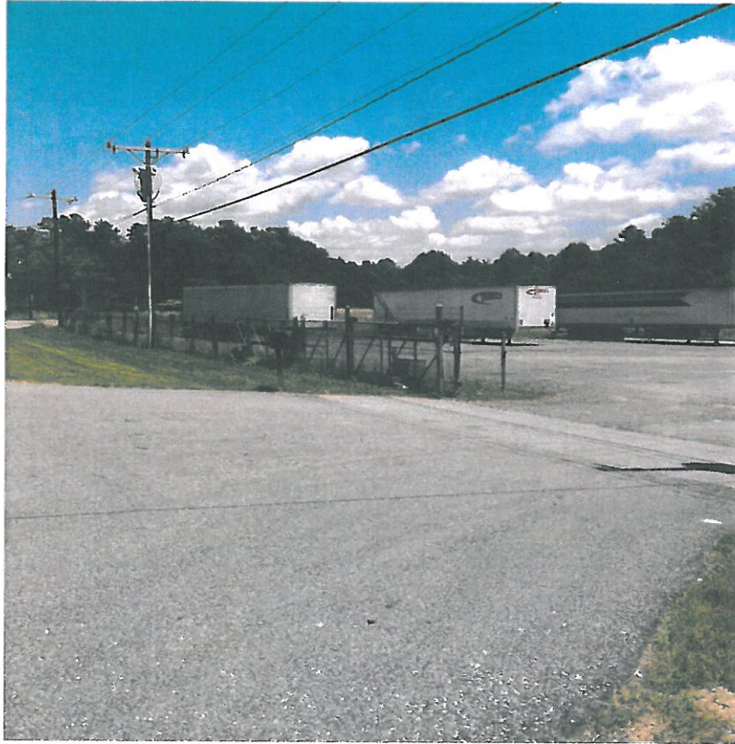
Photograph 3 – View from Elkin Highway looking east.
