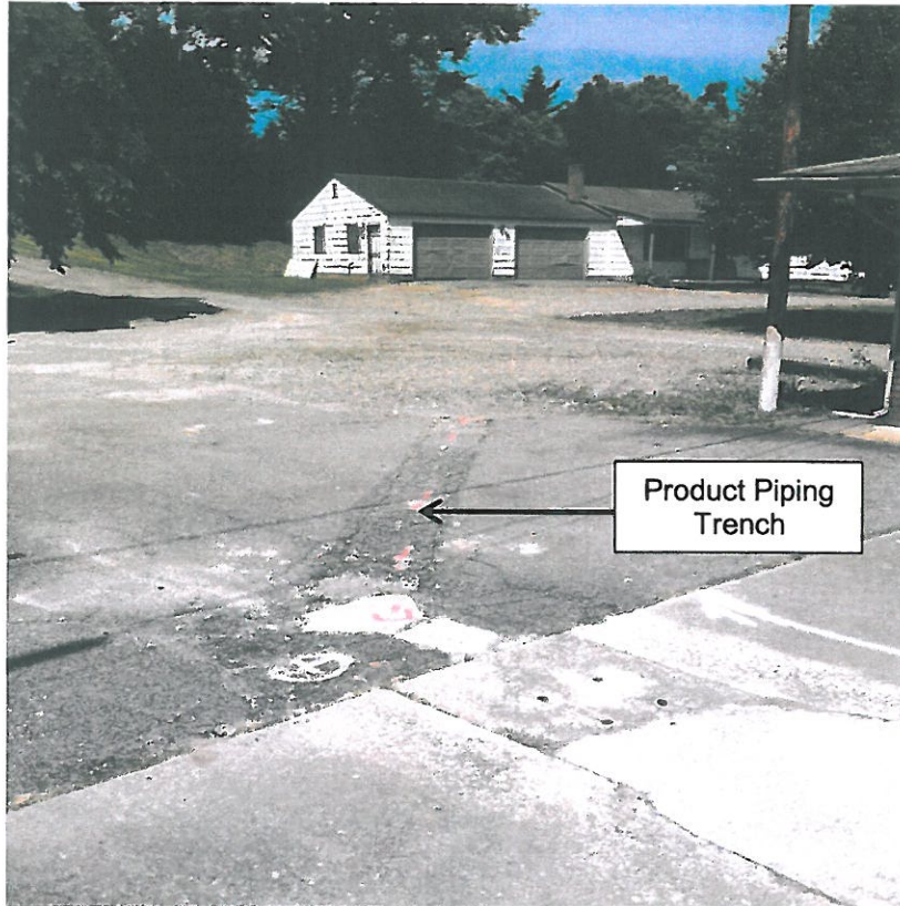
Photograph 5 –View of the product piping trench.
