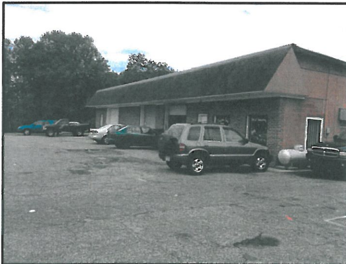
Existing Auto Sales Building (Photograph Facing Approximately Southeast)
