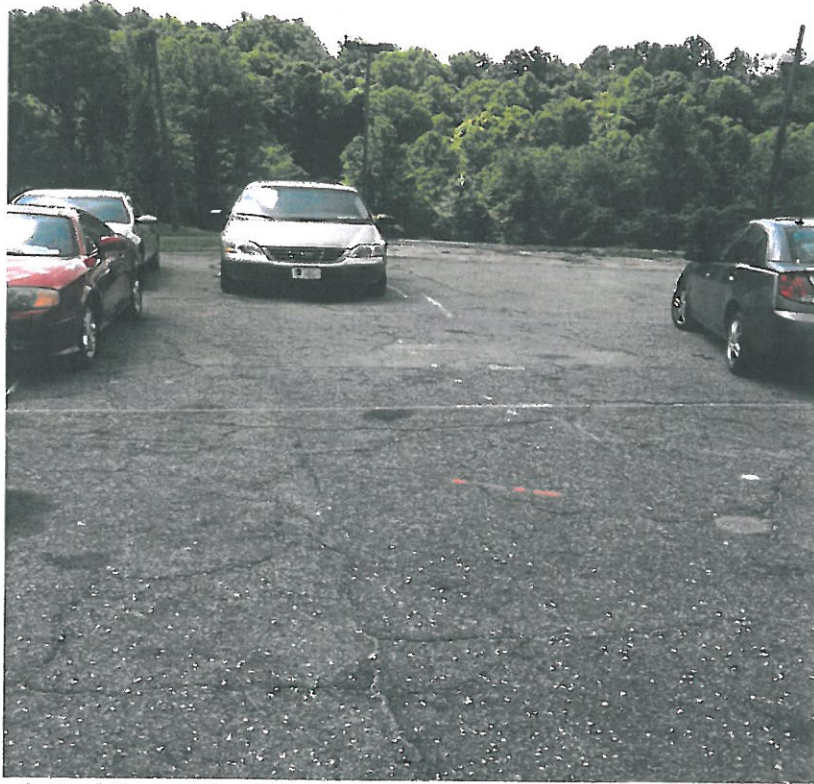
Photograph 3 – View of the USTs located on the western portion of the property.
