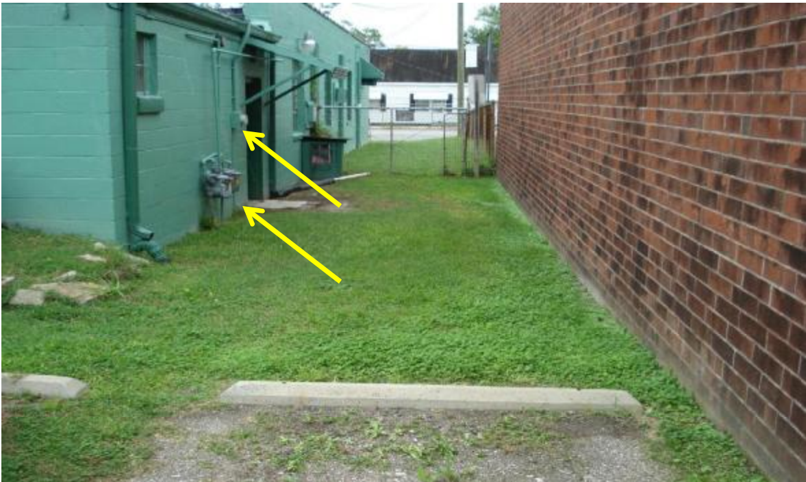
Gas meters and electric lines between buildings at rear of Parcel 174
