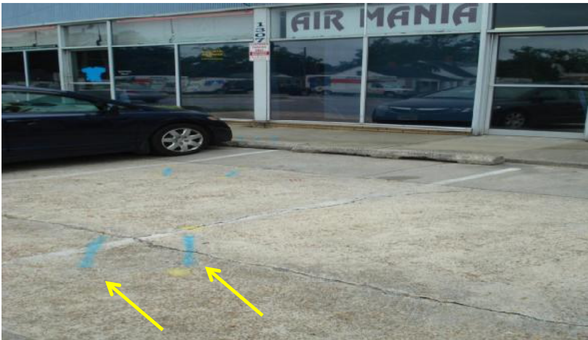
Parallel water service lines to building. Building face off of West 14 th Avenue
