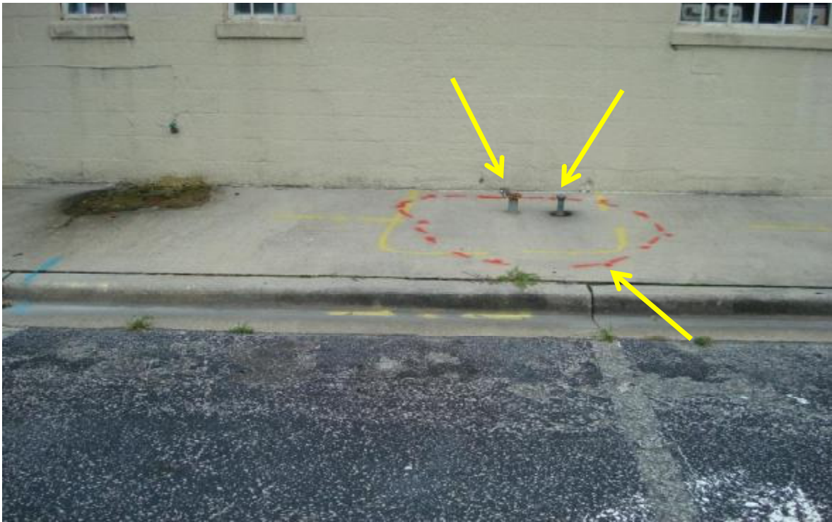
Known UST shown with two metal vents physically on Parcel 49
