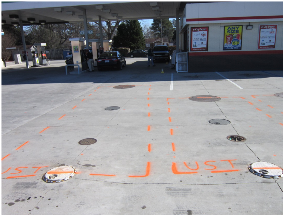
Parcel 129 (Marie S. Williams Property), looking east. Photo shows approximate marked locations of Known UST Nos. 4 and 5 (shown from right to left respectively) near southernmost structure on Parcel 129.
