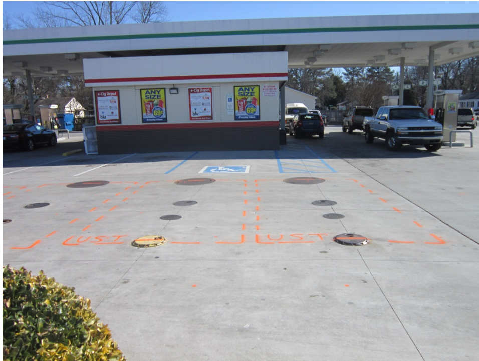
Parcel 129 (Marie S. Williams Property), looking east. Photo shows approximate marked locations of Known UST Nos. 1, 2, and 3 (shown from right to left respectively) near southernmost structure on Parcel 129.
