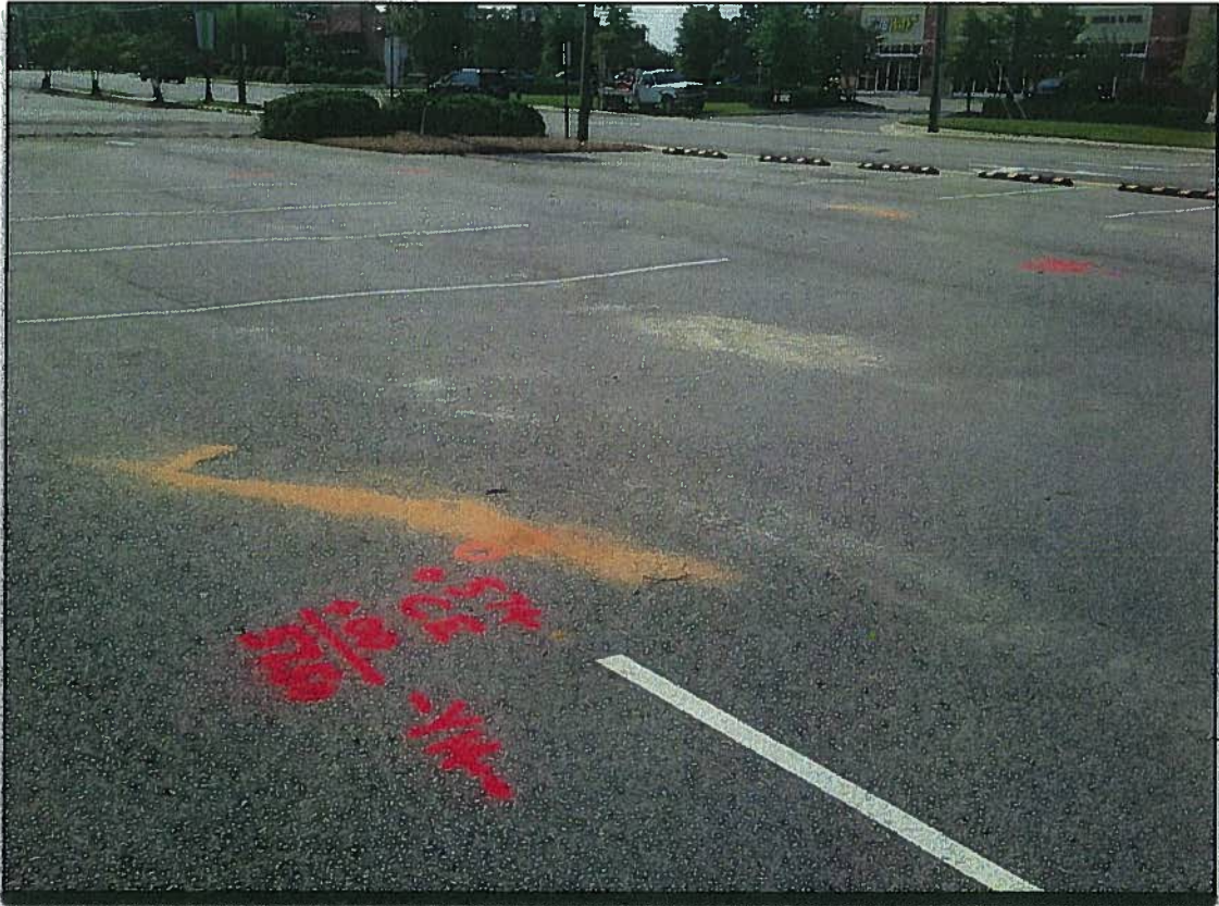
From near Evans Street looking South-southeast.
