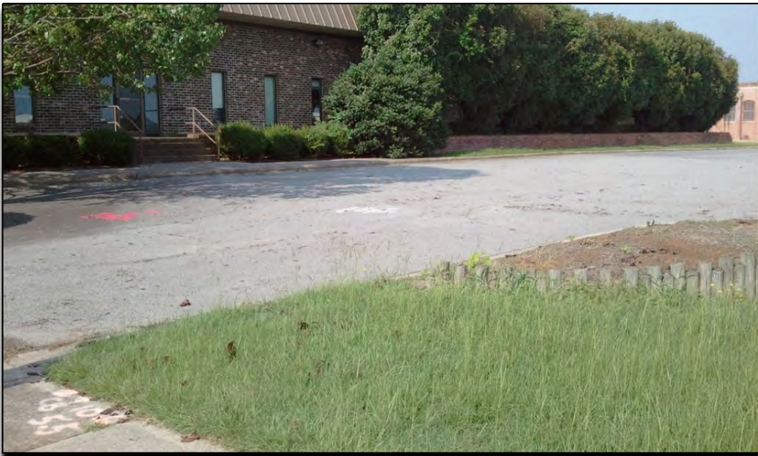
From near corner of W. 10th St. and S. Washington St. looking Southwest across site, proposed catch basin number 1016 (DPT-02) location in left foreground.
