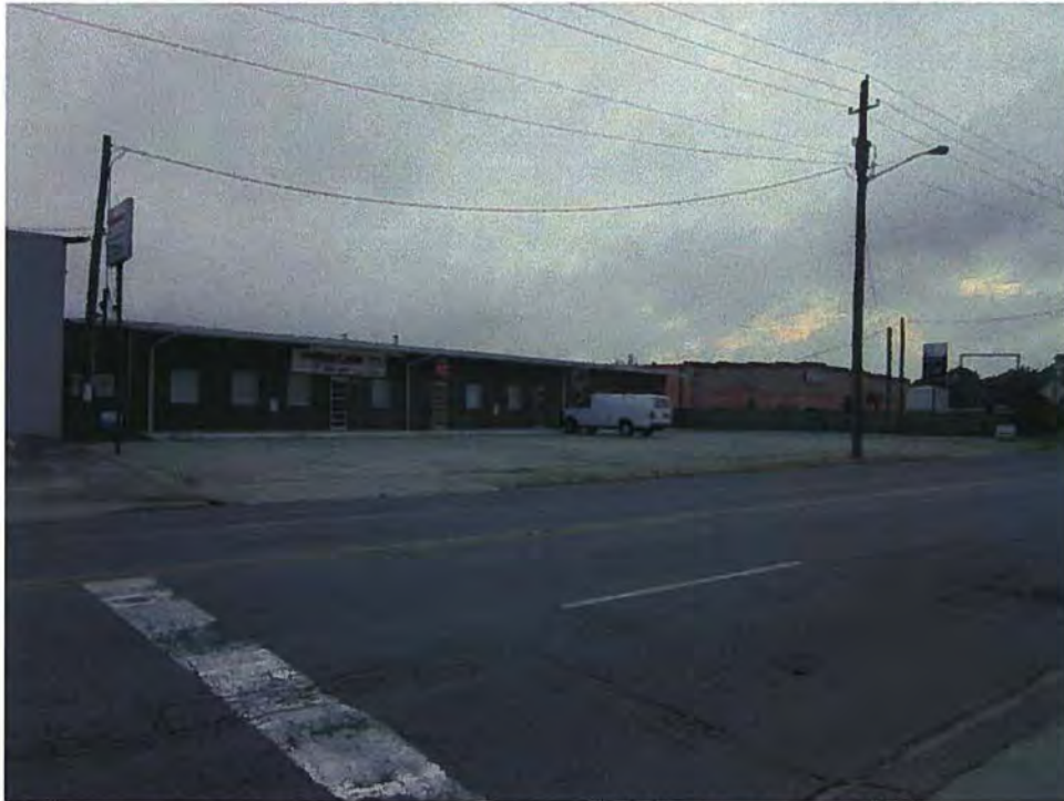
Parcel 93 (Sam Pollard and Son Property), looking northeast
