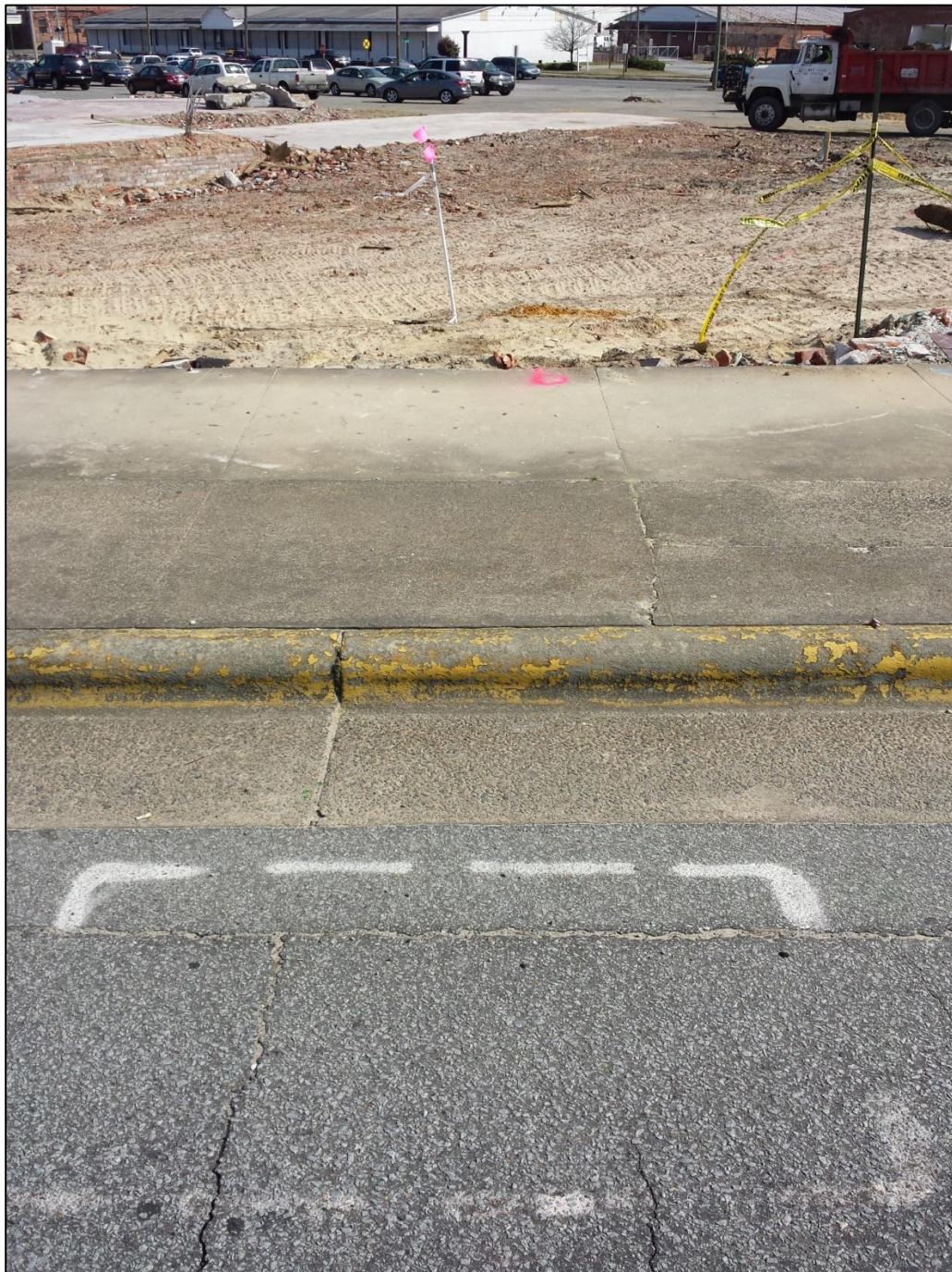
From Dickinson Ave. north of the site looking southwest across site. Geophysical anomaly (suspected UST) outlined with white paint on street in foreground. Soil sample 87-HA-09 (2') location indicated at edge of sidewalk with pink spray paint (upside down number 9). Temporary well 87-TMW-01 with pink flags atop PVC riser.
