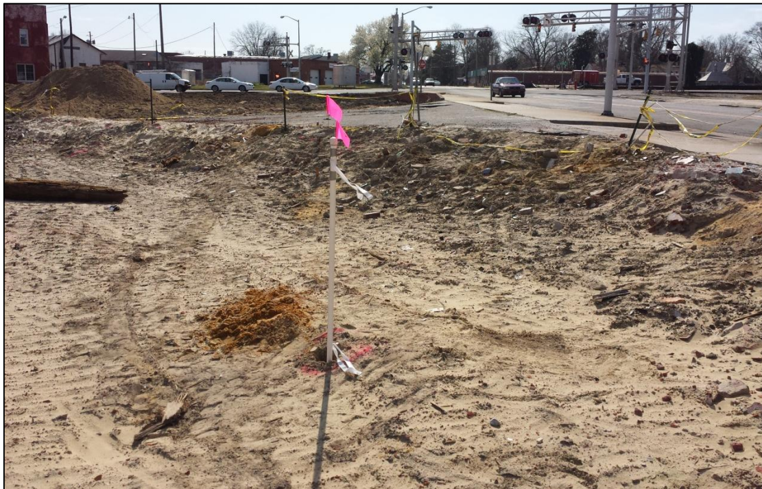
From near northeast property corner looking west along the northern property line. Temporary well (87-TMW-01) located along proposed drainage line.
