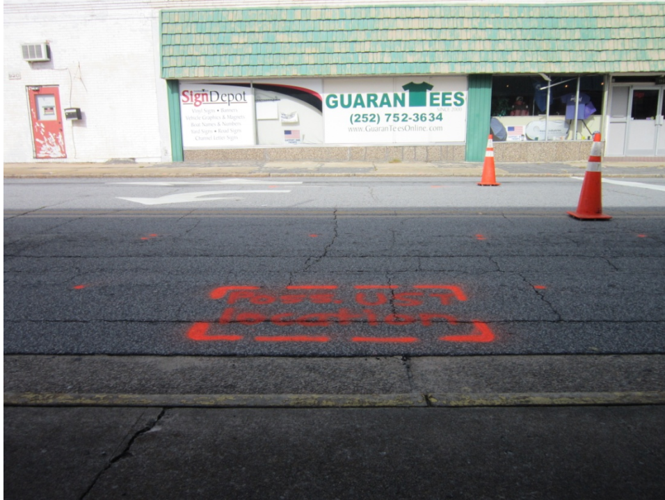
Parcel 87 (First South Bank Property), looking northwest. Photo shows approximate marked location of Possible UST No. 1 near the northern edge of the parcel.
