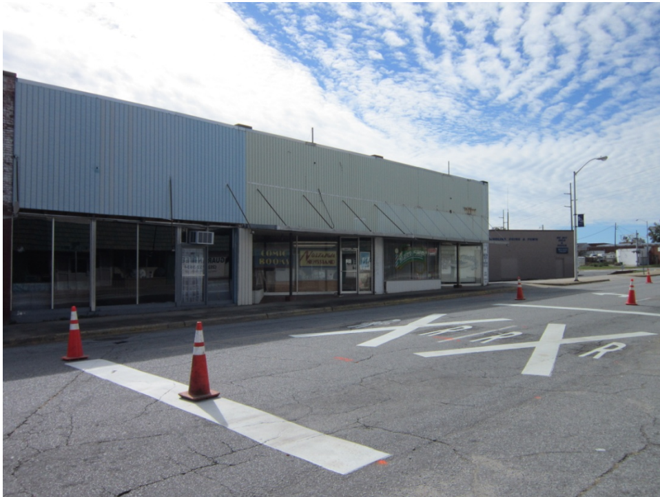
Parcels 85 & 87-91 & 911 Dickinson Ave. (Various Properties), looking south
