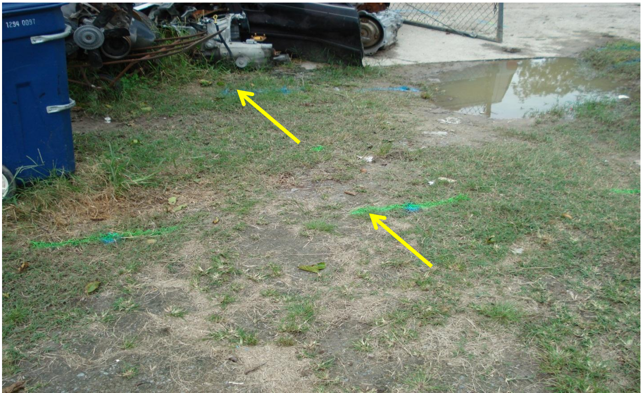
Unknown utility marked in blue and Sanitary Sewer marked in green
