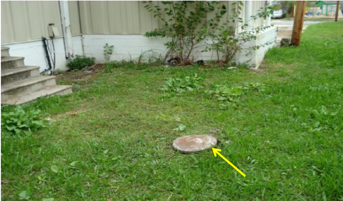
Probable UST propane tank with gas service to building
