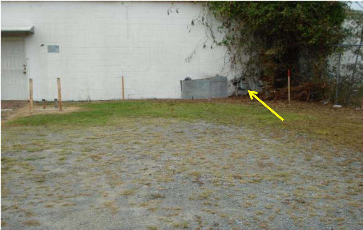
BACK OF BUILDING GAS METER ON RIGHT SIDE AND SERVICE TO BUILDING
