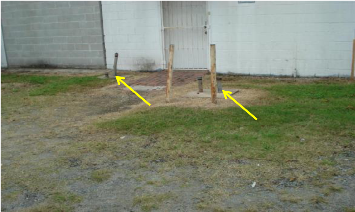
PHOTO SHOWING VENTS FOR PROBABLE UST'S ON BACK SIDE OF BUILDING EITHER SIDE OF DOOR
