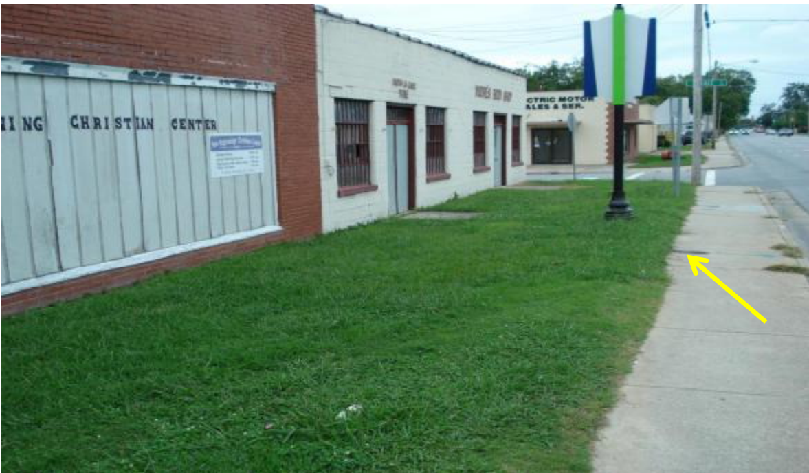
FRONT OF BUILDING SHOWING WATER METER AND SERVICE TO BUILDING
