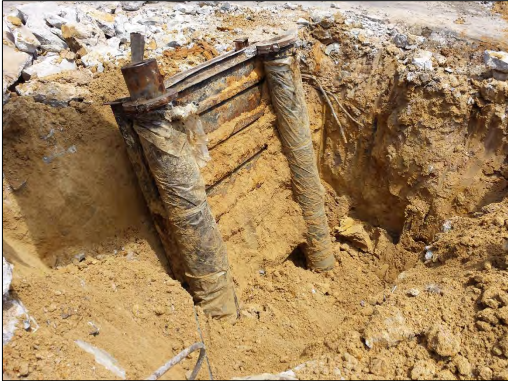
Dual post hydraulic lift excavation.
