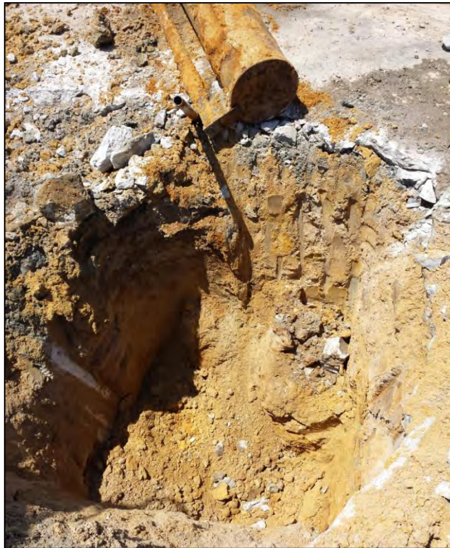
Removed single post hydraulic lift.
