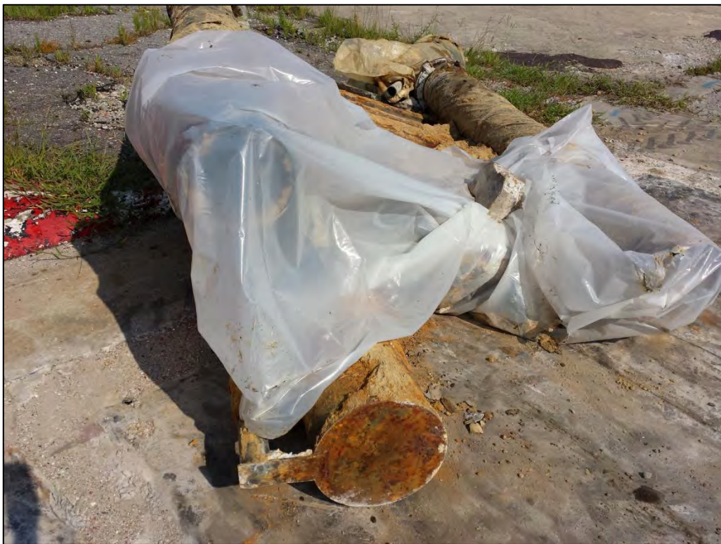
Removed hydraulic lift cylinders.
