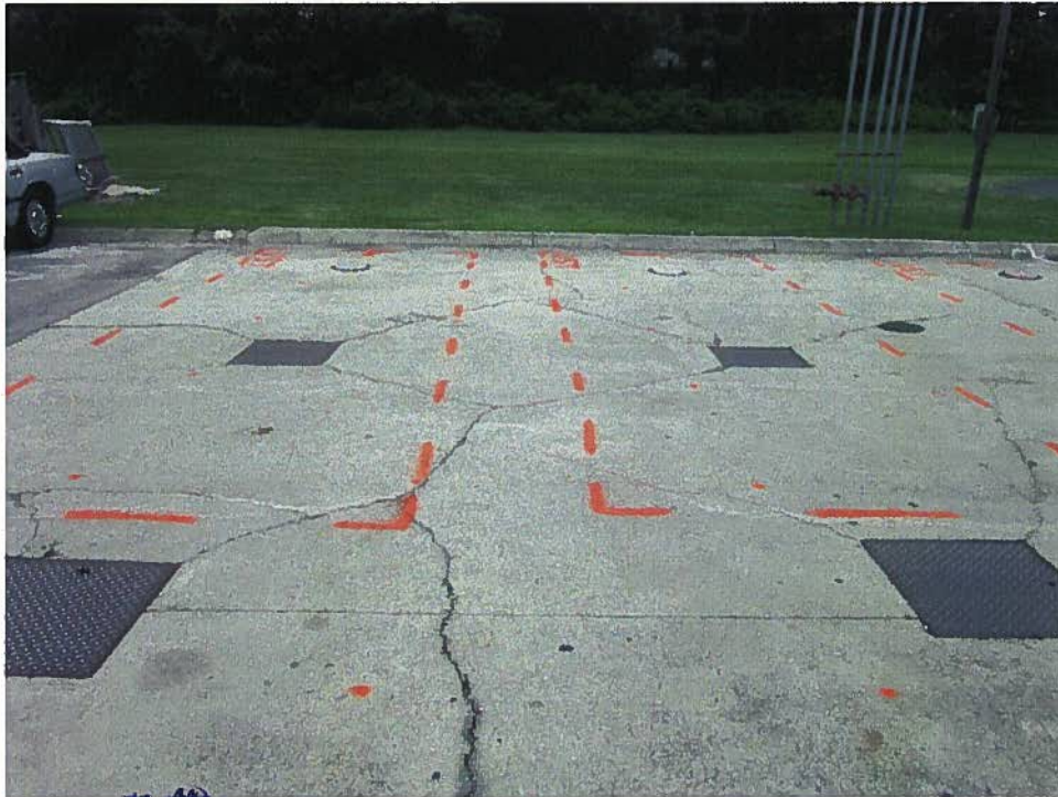
Parcel 48 (RI CS5, LLC Property), looking north. Photo shows approximate marked location of known UST Nos. 1 and 2 near the northwest corner of the building.
