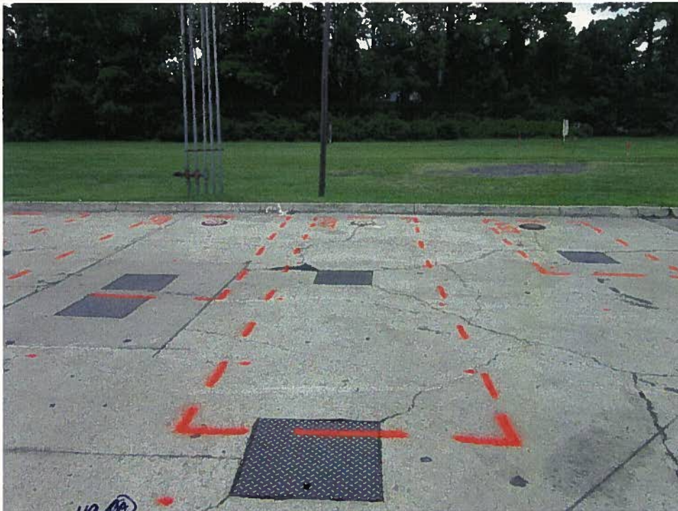
Parcel 48 (RI CS5, LLC Property), looking north. Photo shows approximate marked location of known UST Nos. 3, 4, and 5 near the northeast corner of the building.
