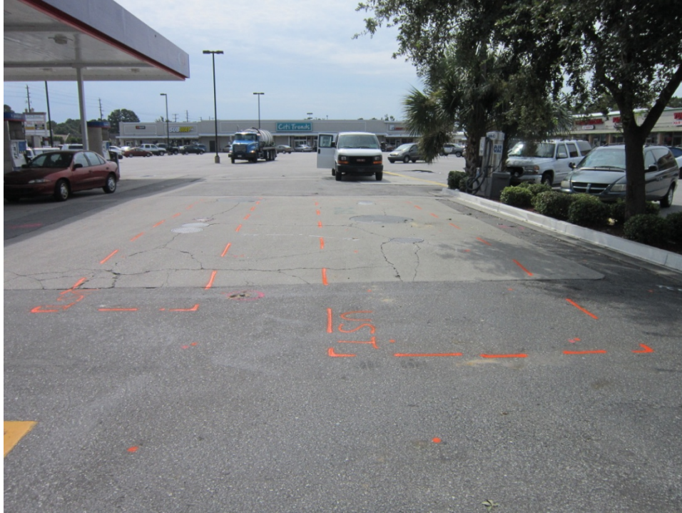
Parcel 51 (RI CS5, LLC Property), looking south. Photo shows approximate marked location of known UST Nos. 1 and 2 near the northwest corner of the parcel.
