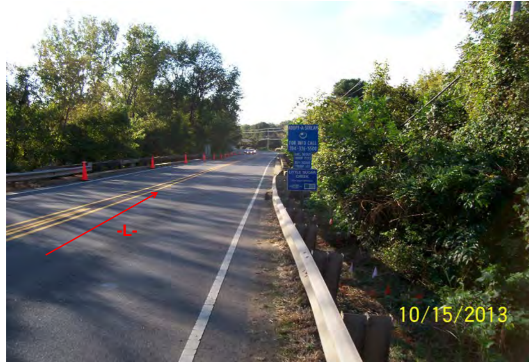
View Looking Upstation along -L- from End Bent 1
