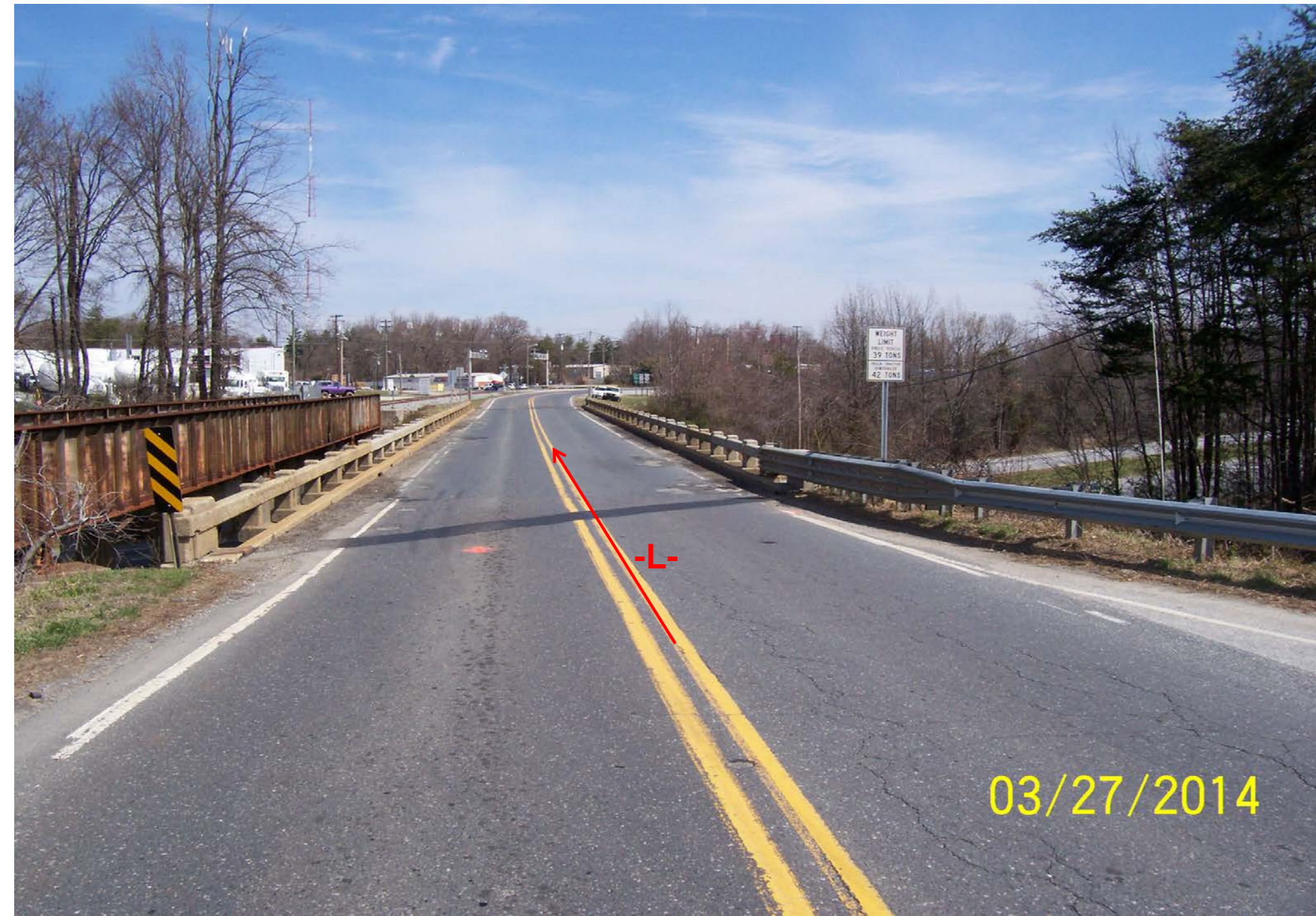
View Looking North along -L- from End Bent 1
