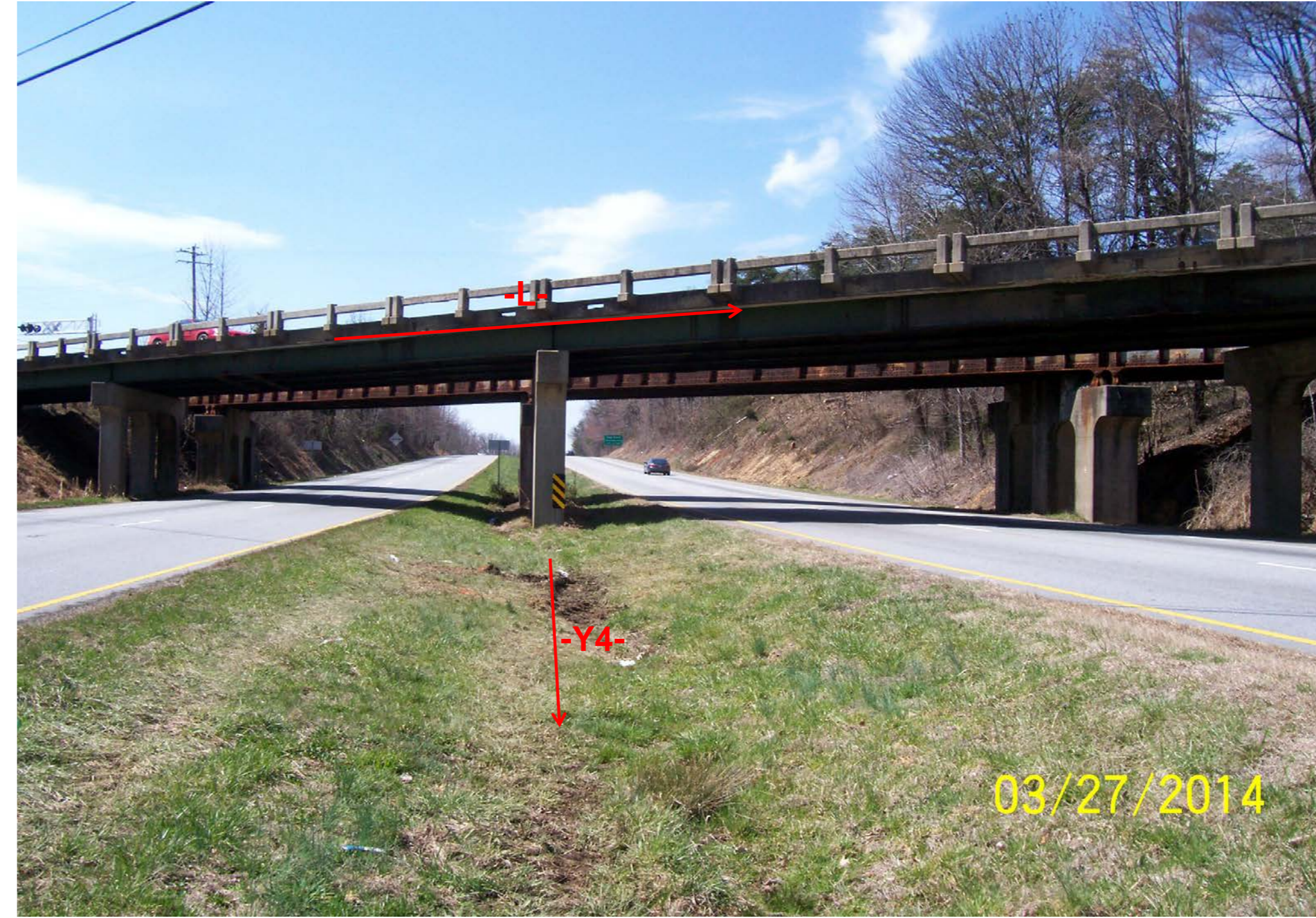
Profile of Bridge From B1-B Looking West
