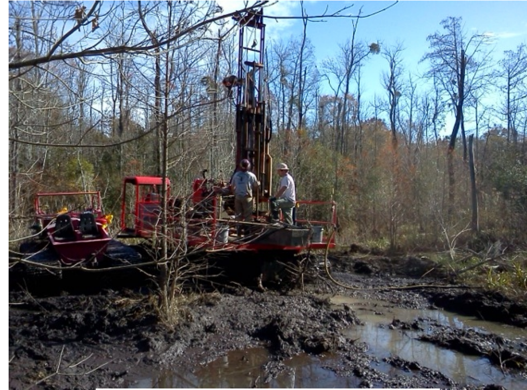
DRILL ON BORING B-11A SBL FACING NORTH ALONG -L- SBL
