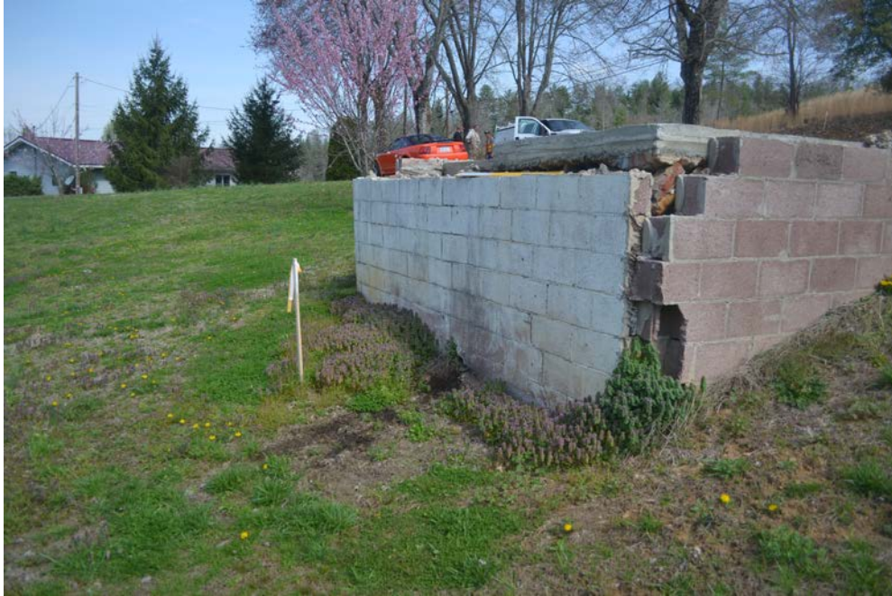
Photograph 4: View of southwest exterior of oil change pit at the site. Oil stained grass can be seen emanating from an outlet drain from the base of the oil change pit. A NCDOT ROW stake can be seen in foreground.
