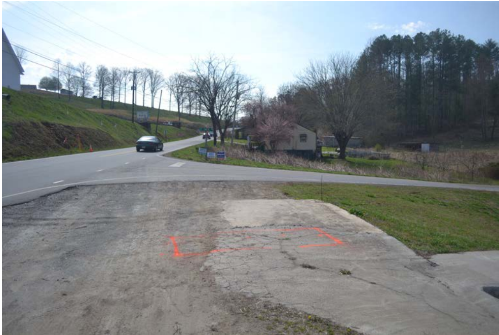
Photograph 1: Potential UST (4' by 8') identified at NCDOT Parcel 23 by GPR and demarcated in orange paint on April 4, 2014. View is to the southeast parallel to NC 294. Crowe Road can be seen to from left to right in background.
