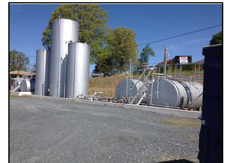
View of North Portion of Survey Area & ASTs (Facing Approximately Northwest)
