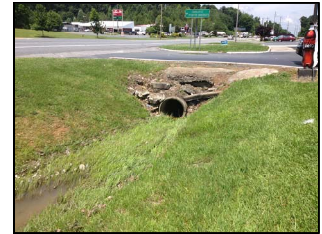
Photo #1: Drainage pipe extending under east driveway entrance
