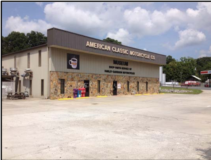
View of Main Building (Facing Approximately Northeast)
