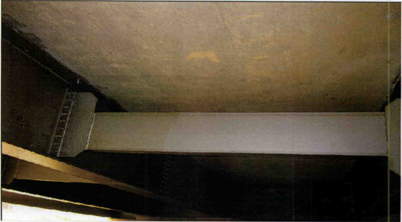
SUPERSTRUCTURE OF SPAN 1
