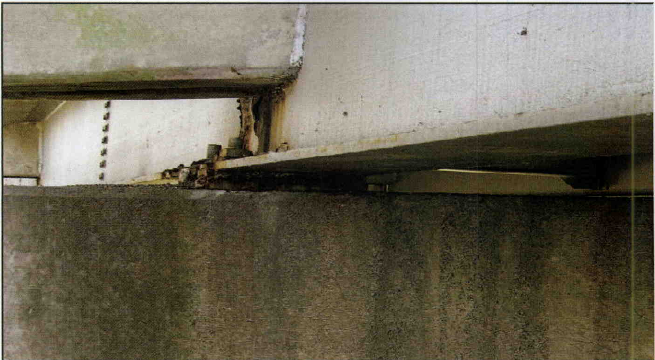
BEARING AT LEFT SIDE OF BENT 1
