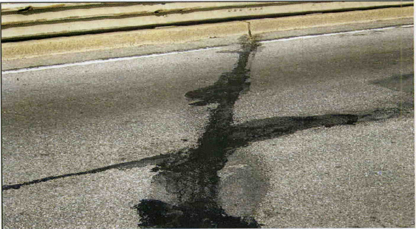
ASPHALT WEARING SURFACE OVER BENT 4 OTHERS SIMILAR
