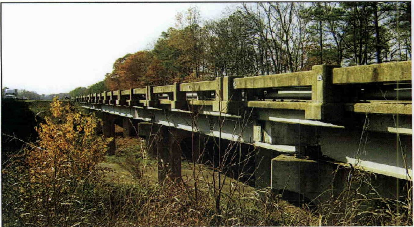
EAST SIDE LOOKING WEST
