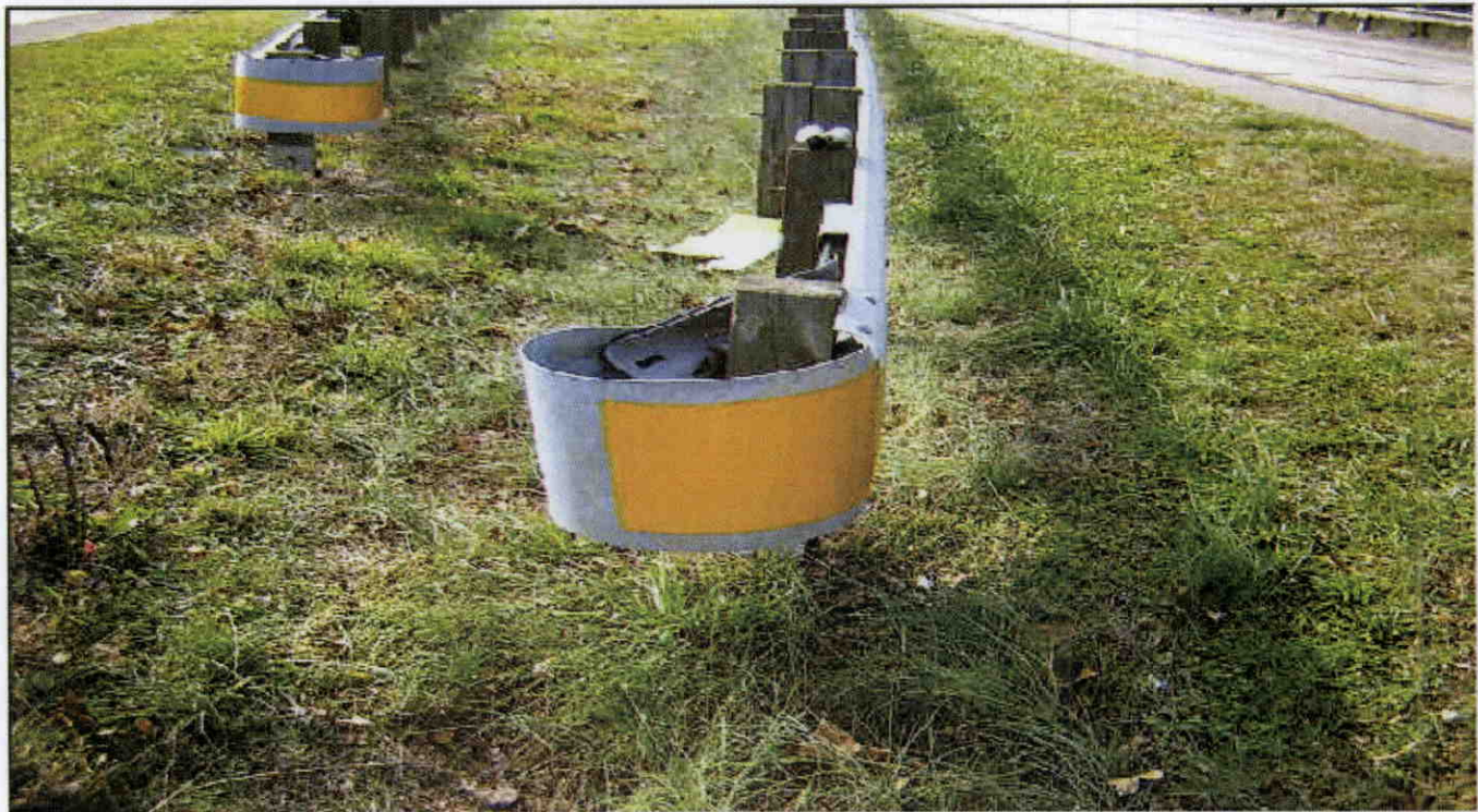
RIGHT GUARDRAIL TERMINAL AT APPROACH 2
