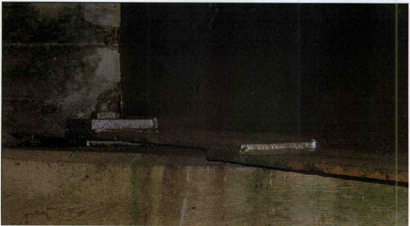
END OF BEAM 1 AT END BENT 1
