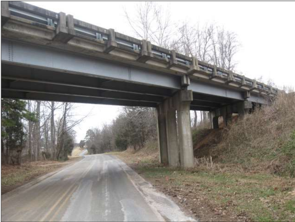
EAST SIDE LOOKING WEST PHOTO 1 OF 2
