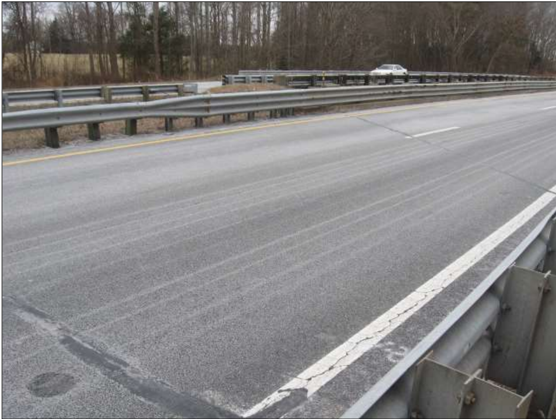
APPROACH ROADWAY @ NORTH END ( SOUTH END SIMILAR )
