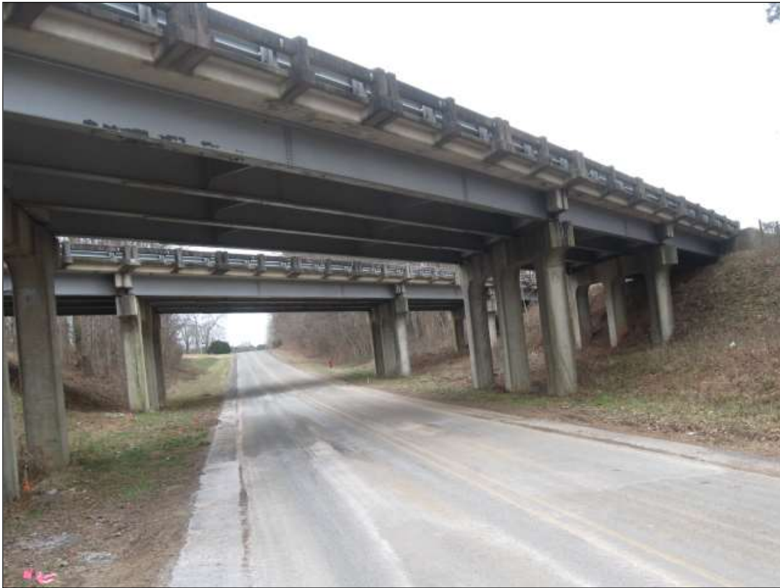
WEST SIDE LOOKING EAST PHOTO 1 OF 2
