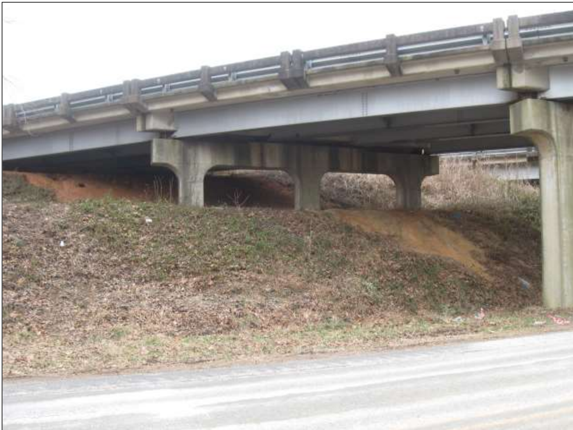
WEST SIDE LOOKING EAST PHOTO 2 OF 2
