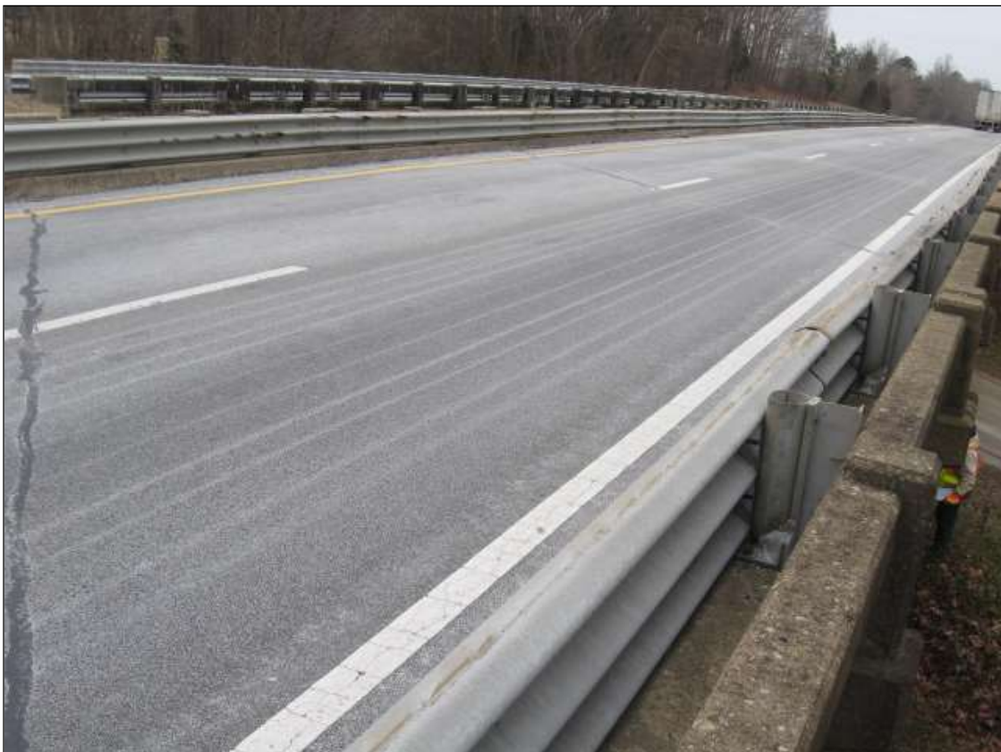
ASPHALT WEARING SURFACE SPAN 5 TOP OF DECK ( ALL OTHER SPANS SIMILAR )
