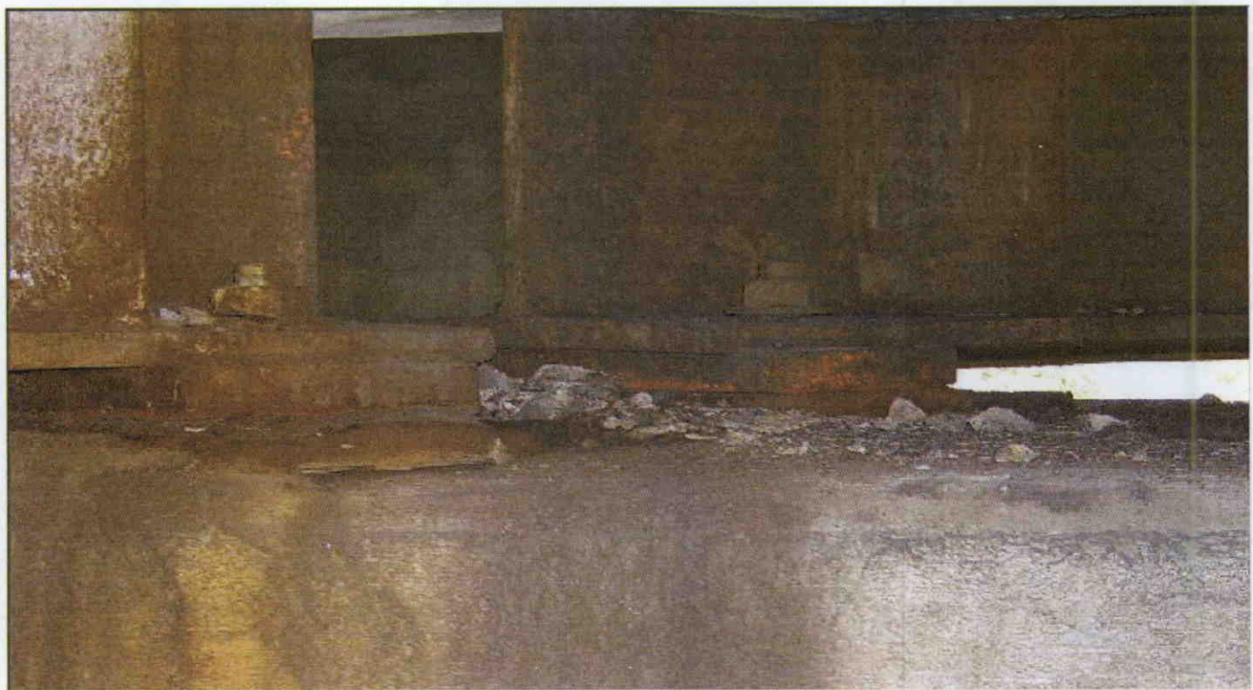
BEARING AT BEAM 2 BENT 1
