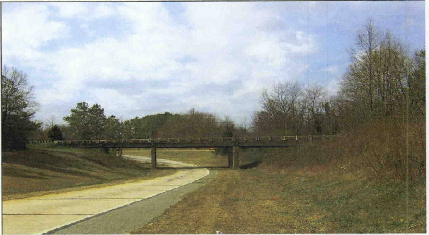
EAST SIDE LOOKING WEST
