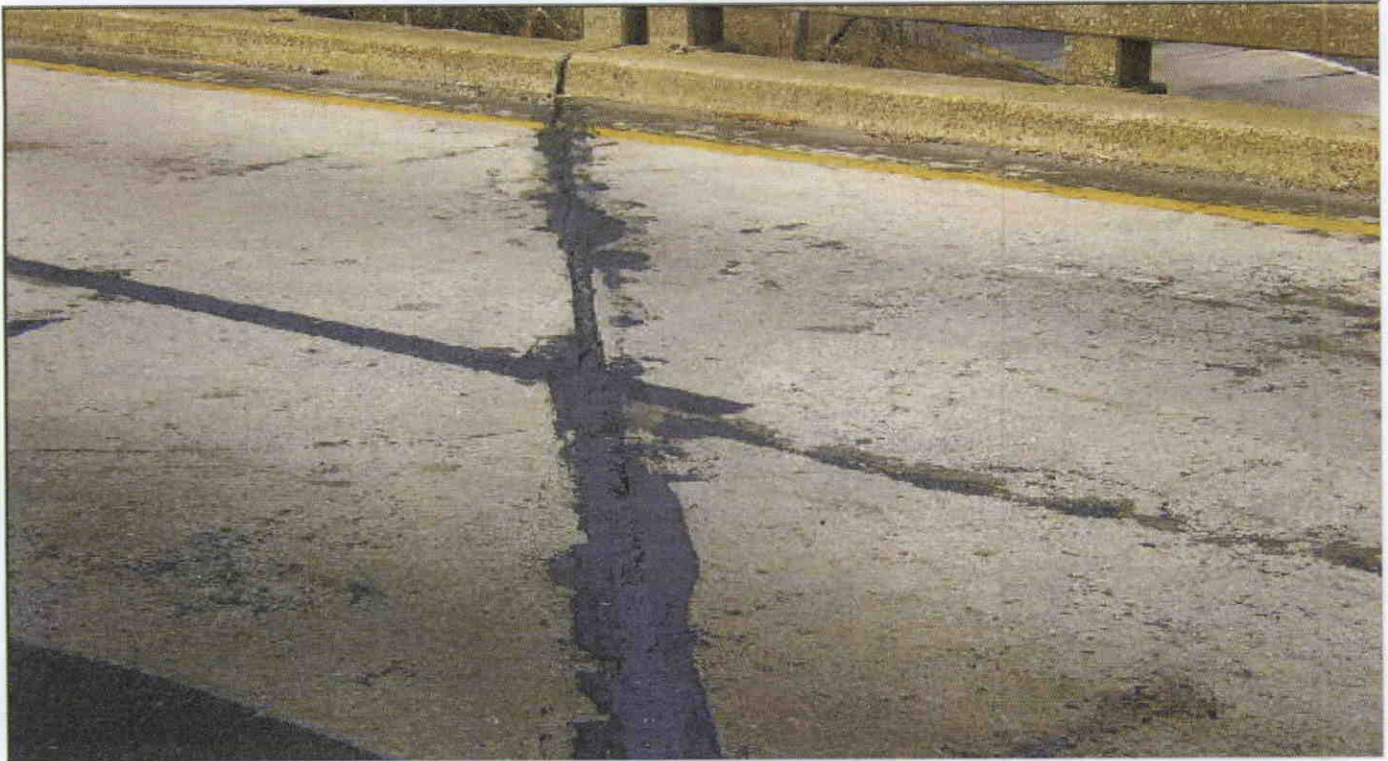
JOINT IN TOP OF DECK OVER BENT 1
