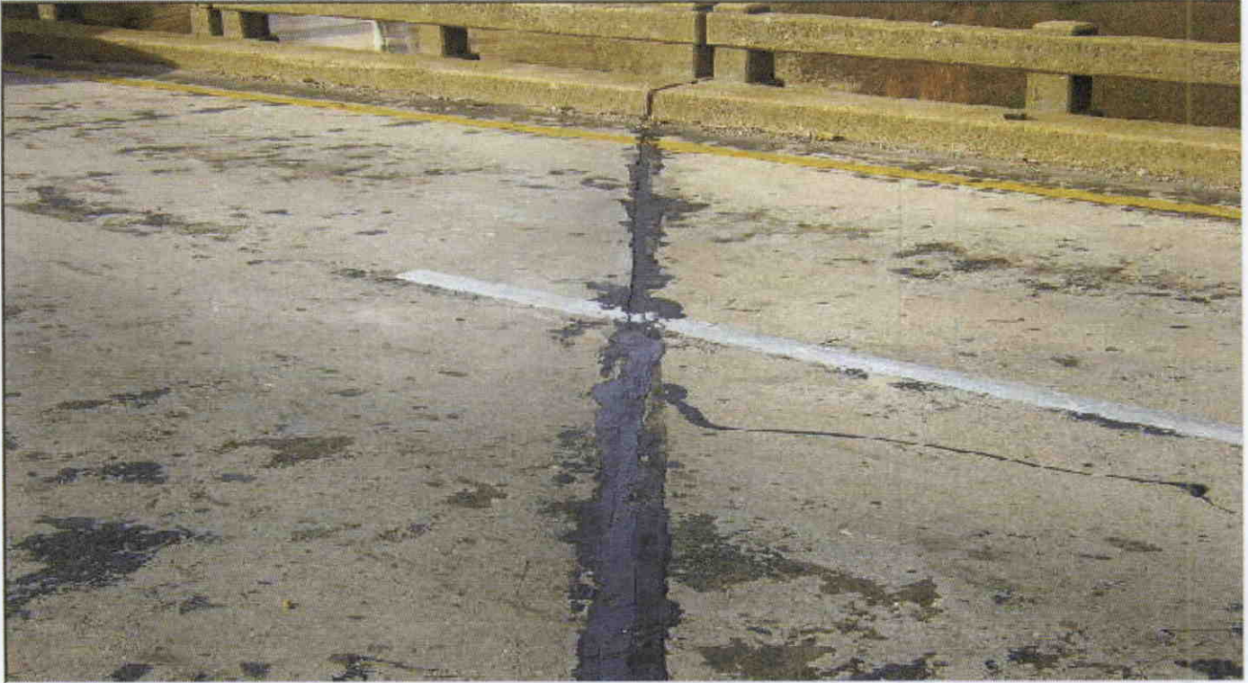
JOINT IN TOP OF DECK OVER BENT 3
