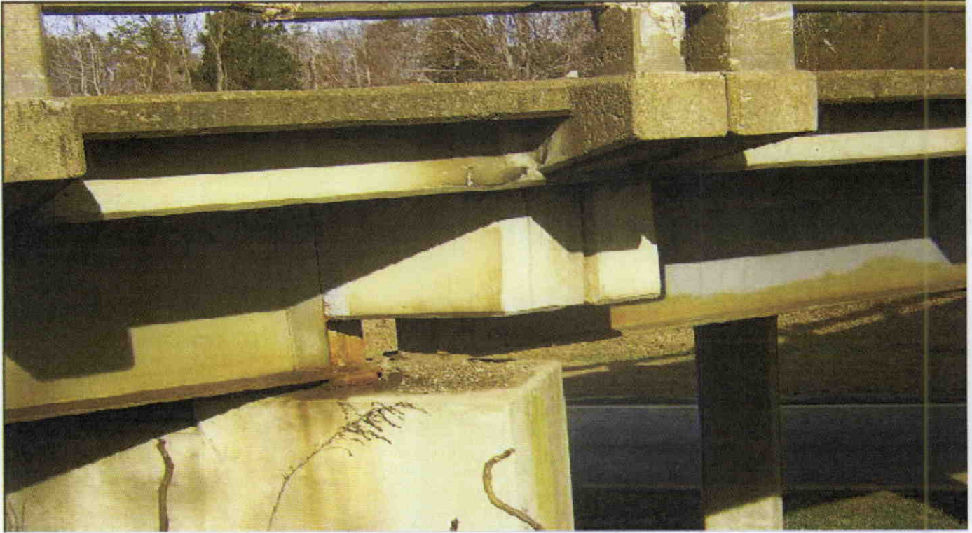
SUPERSTRUCTURE OVER RIGHT SIDE OF BENT 1
