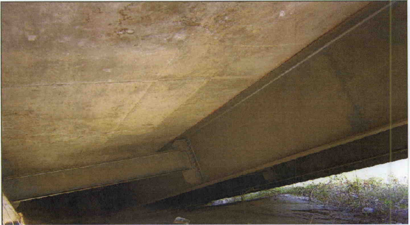
SUPERSTRUCTURE OF SPAN 1
