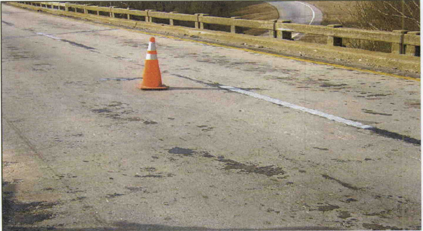
TOP OF DECK SPAN 4
