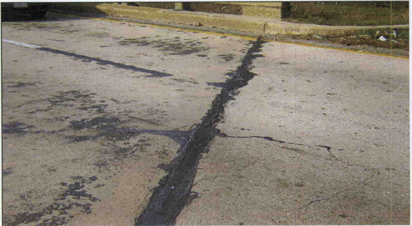
JOINT AT END BENT 2 END BENT 1 SIMILAR
