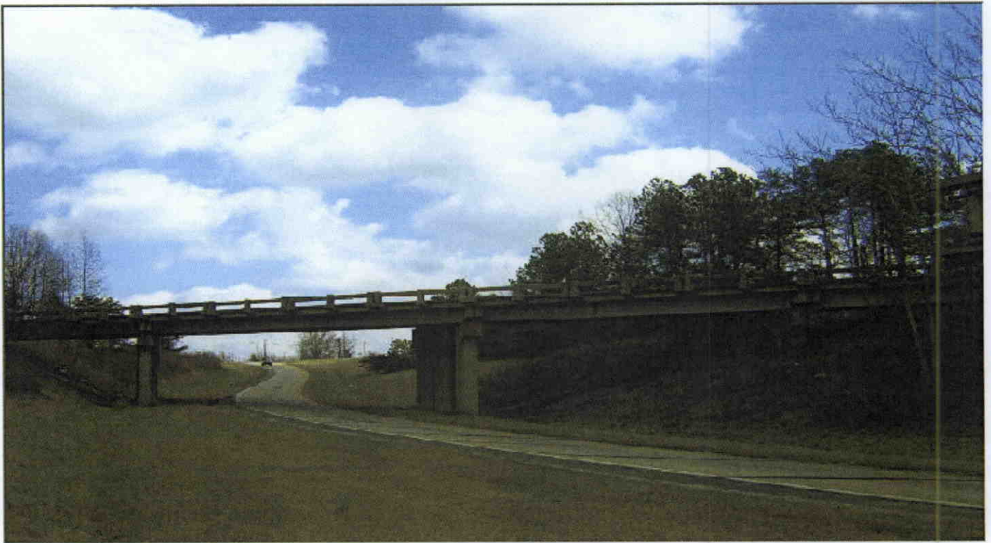
WEST SIDE LOOKING EAST
