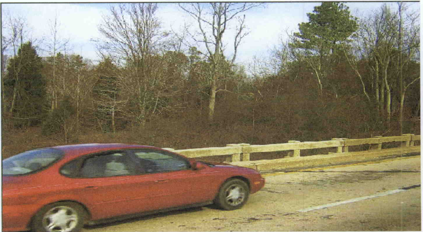
GUARDRAIL REPAIR AT LEFT SIDE OF END BENT 2
