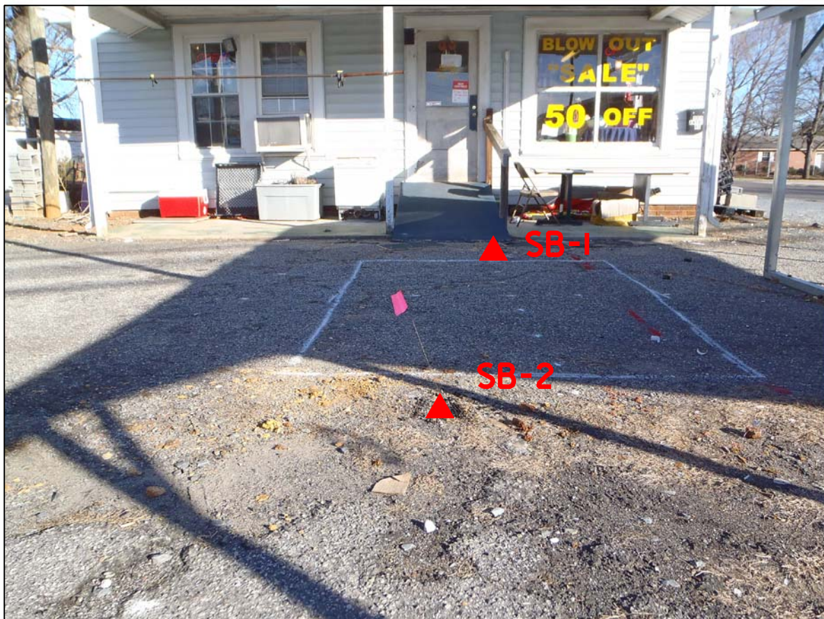
PHOTO 2 - BORINGS AT GEOPHYSICAL ANOMALY LOOKING EAST
