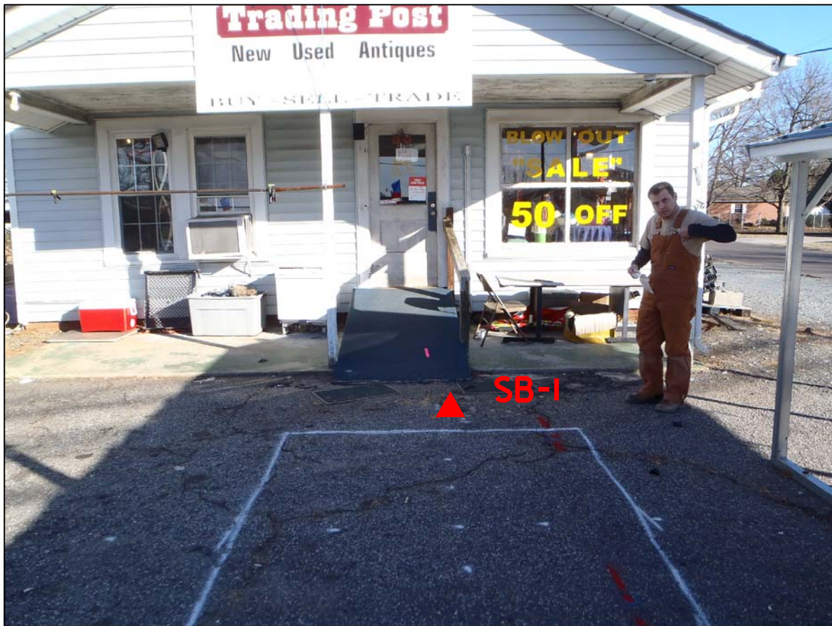
PHOTO 1 - BORING AT GEOPHYSICAL ANOMALY LOOKING EAST
