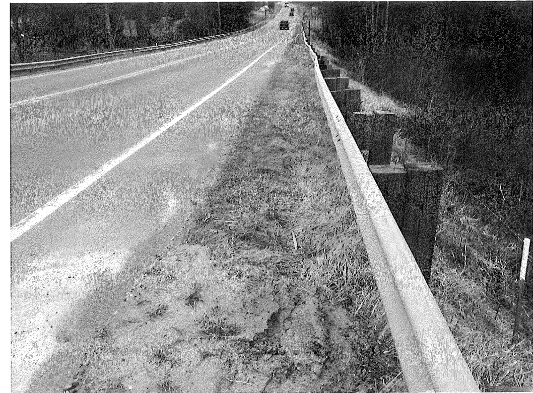
EB2-C Looking Towards EB1-C
