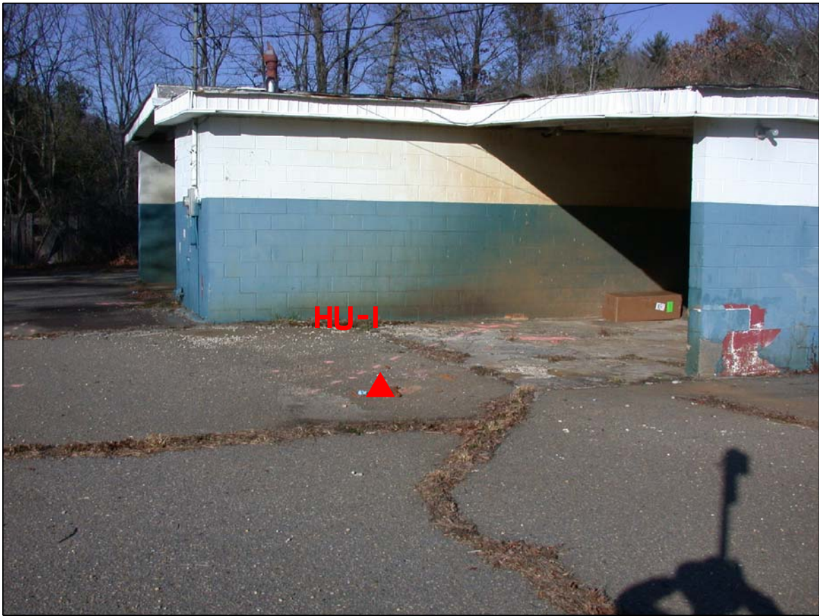
PHOTO 1 - BORING ON WEST SIDE OF CAR WASH LOOKING NORTHEAST
