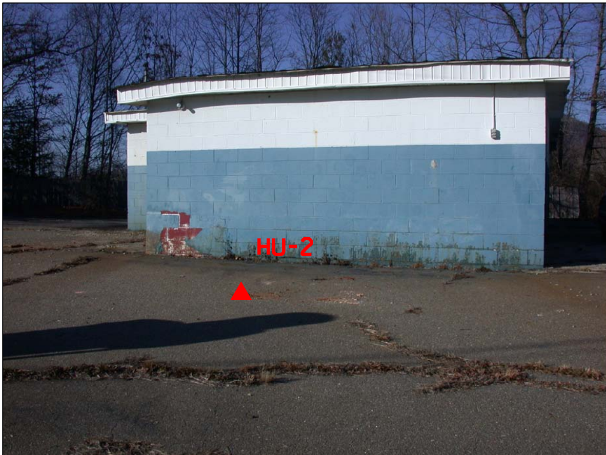
PHOTO 2 - BORING ON SOUTH SIDE OF CAR WASH LOOKING NORTHEAST
