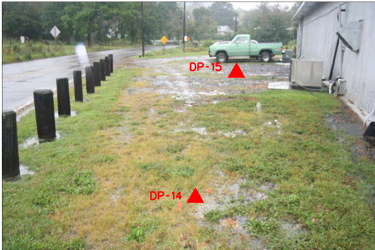
PHOTO 12 - VIEW FROM REAR OF BUILDING LOOKING WEST
