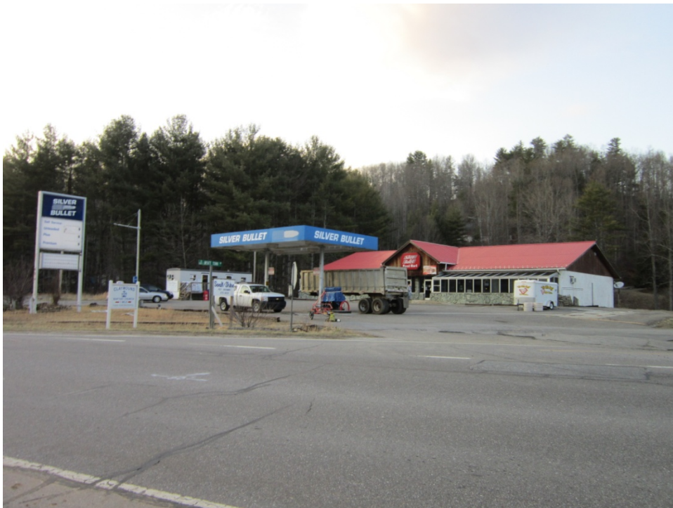
Parcel 12 (William Young Property), looking northwest
