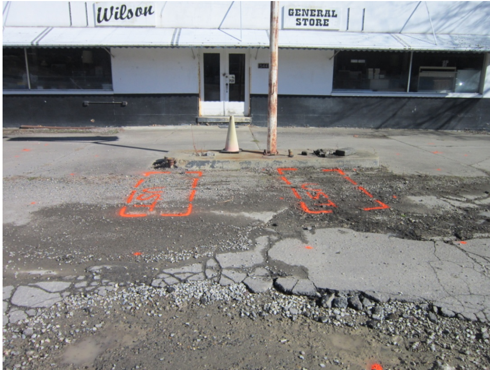
Howell Property, looking northeast. Photo shows marked approximate locations of probable UST Nos. 1 and 2 south of the pump island in front of the former Wilson General Store.
