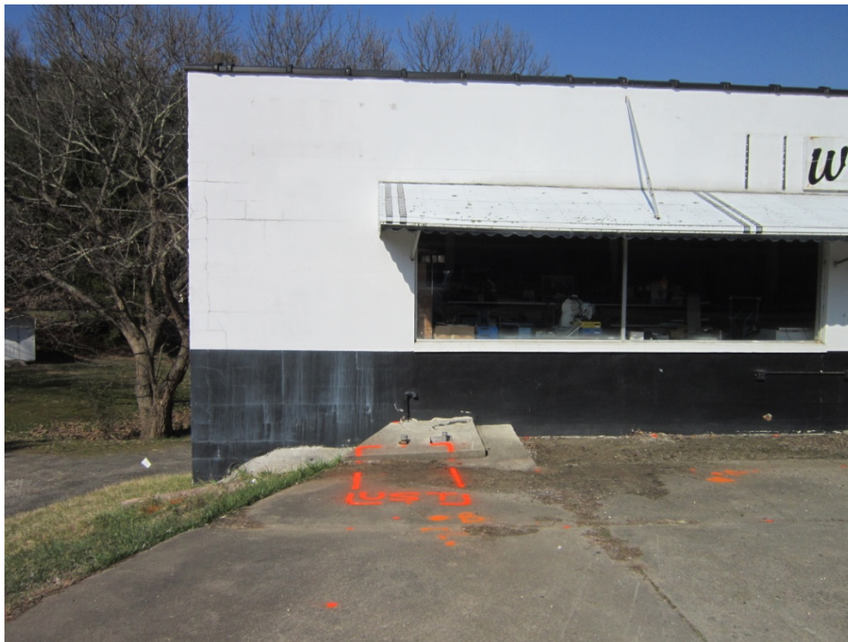
Howell Property, looking northeast. Photo shows marked approximate location of probable UST No. 3 near the southeastern corner of the former Wilson General Store.
