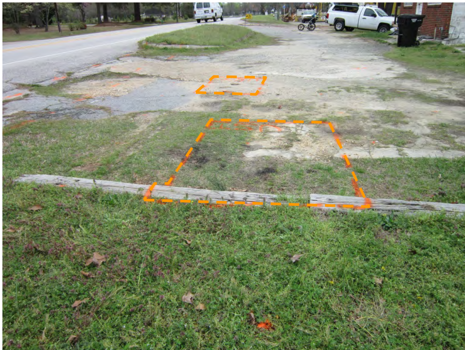
Parcel 14 (Richard Hillman Property), looking northeast. Photo shows approximate marked locations of Probable UST Nos. 1 and 2 near the northern end of Parcel 14.
