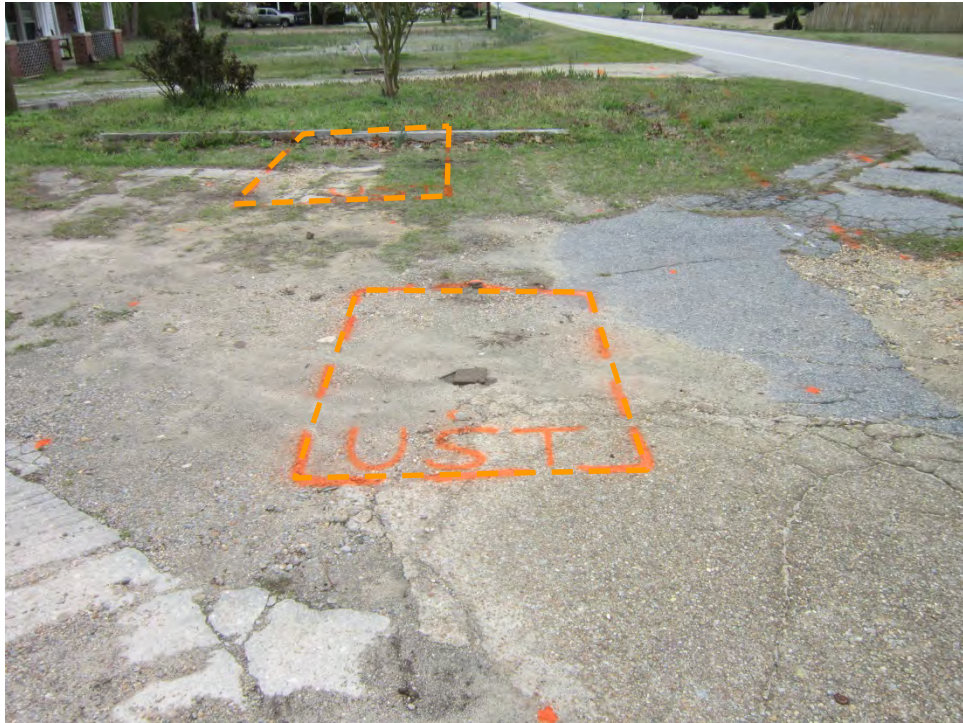
Parcel 14 (Richard Hillman Property), looking southwest. Photo shows approximate marked locations of Probable UST Nos. 1 and 2 near the northern end of Parcel 14.
