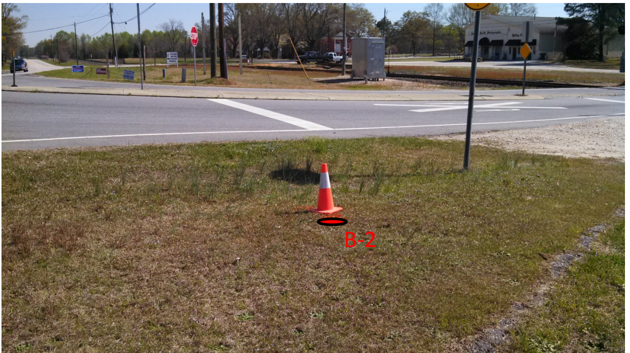
Photo #4: Boring location B-2, facing northeast.
