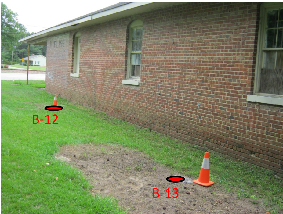
Photo #4: Boring locations B-12 and B-13, facing southwest.
