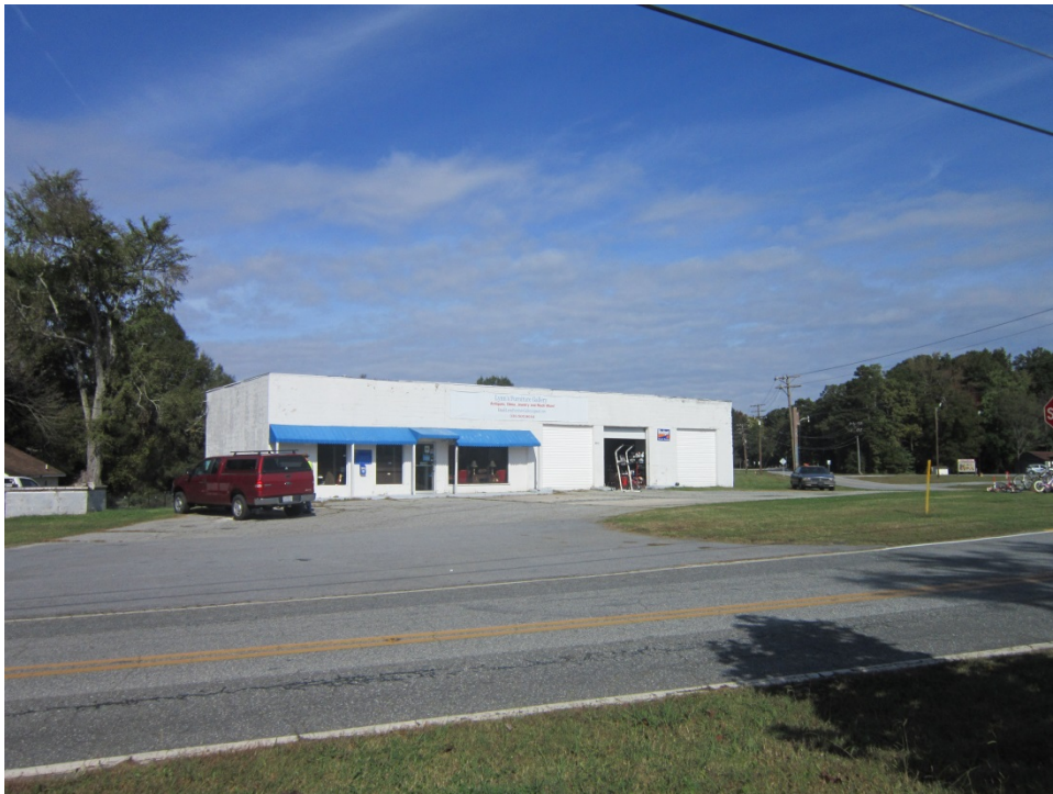
Parcel 17 (Charles & Martha Terry Property), looking northwest
