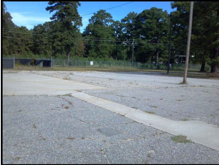
1 Parcel #006 looking northeast.
