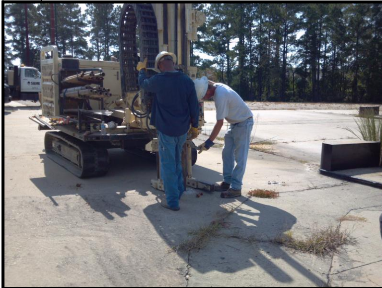
7 Advancing boring near former dispenser island.
