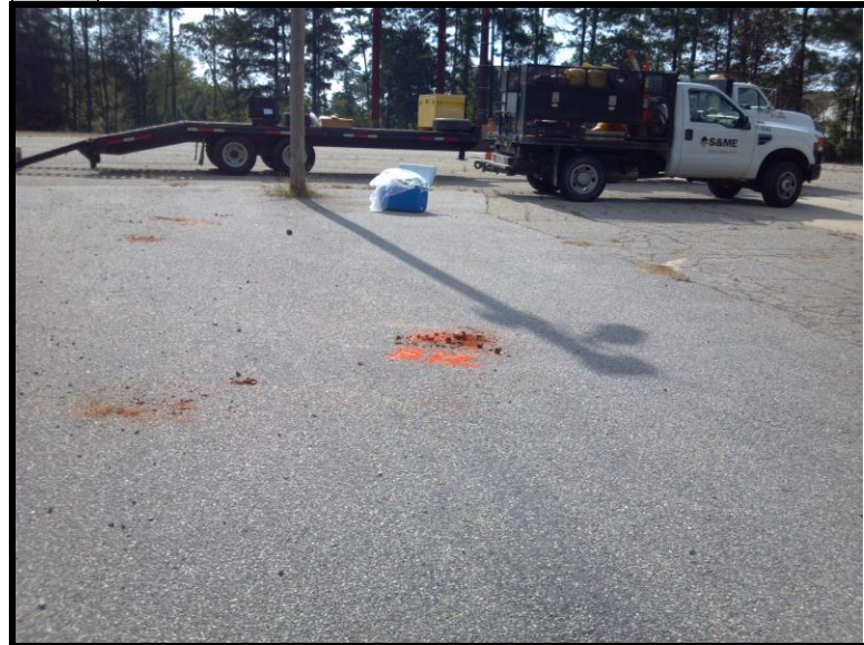
8 Boring B-12 in suspected UST basin. Note the newer asphalt covering the suspected UST basin.
